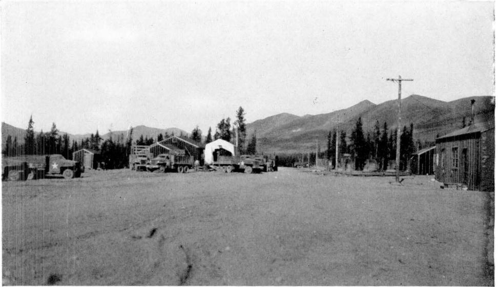
Canol pipe-line road at Pump station No. 10, 78 miles east of Johnsons Crossing, Yukon. Photo by J. S. Stewart, Geological Survey, 1944 (94989).
