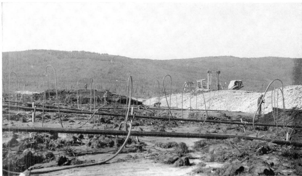
Modern cold-water thawing plant and dredging operations below Granville on Dominion Creek, Klondike placer mining district, Yukon. Photo by H. S. Bostock, Geological Survey (79314).
