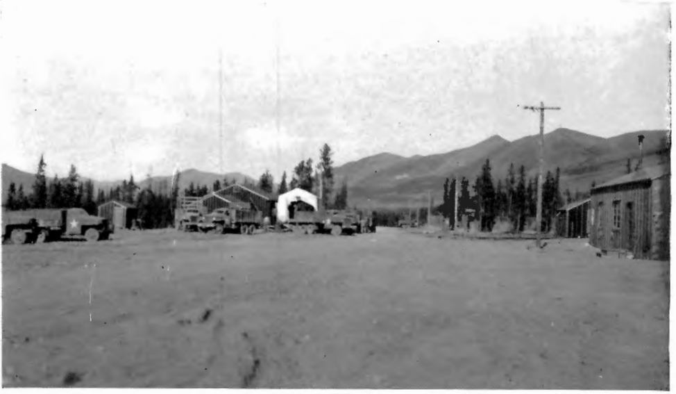
Canol pipe-line road at Pump station No. 10, 78 miles east of Johnsons Crossing, Yukon. Photo by J. S. Stewart, Geological Survey, 1944 (94989).
