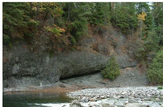
Figure 14. Cretaceous sandy conglomerate and sandstone dip to the south (downstream and to the left in the photograph) and form the support to the west abutment of the Capilano River Bridge of Highway 1.
