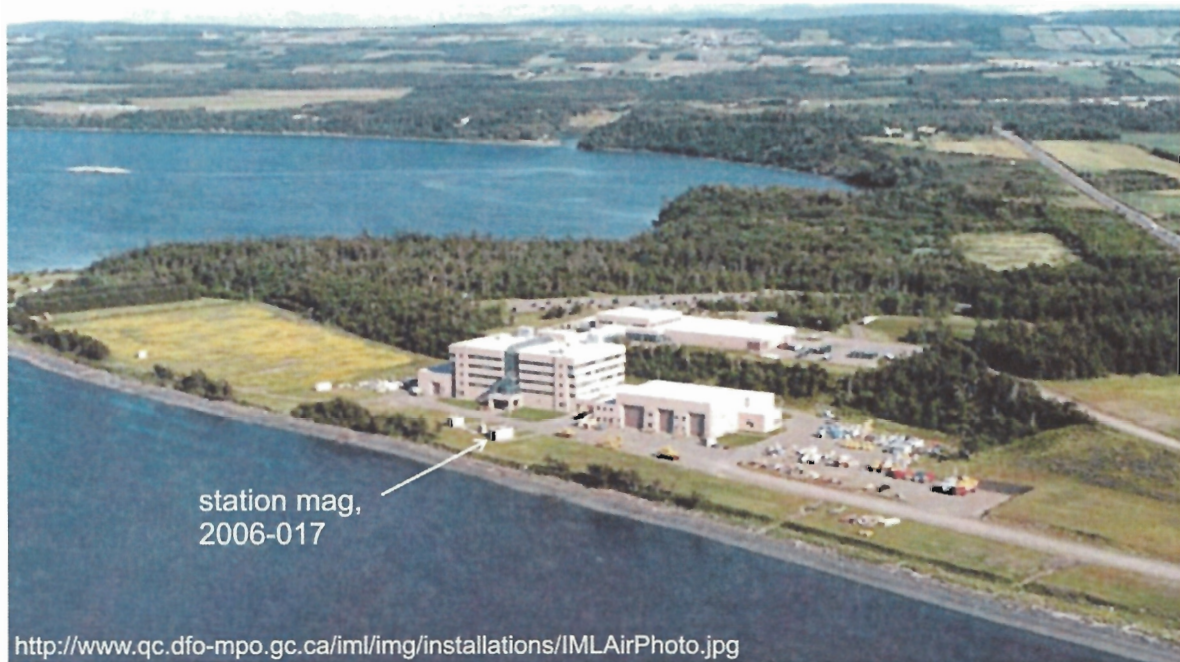
Figure 14- Station magnetometer setup location on the IML campus for this survey.
