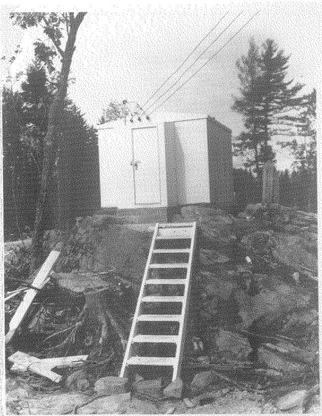
One of the portable seismic huts of the rockburst travel-time project. The hut is set up at La Cave, Quebec, where mains power was available. Normally operation was powered by storage batteries.
