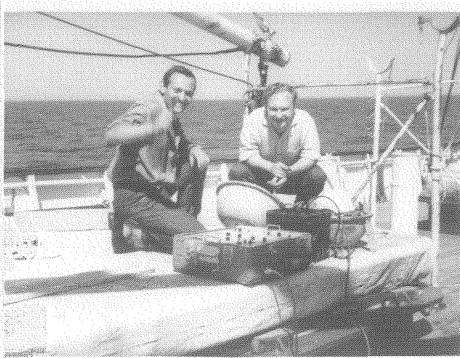
H.D. Valliant, right, with the underwater gravimeter and its water-tight case.
