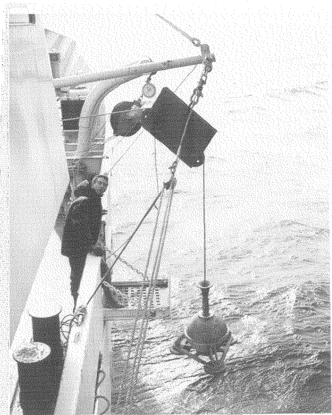
The underwater gravimeter about to be lowered to the ocean floor.
