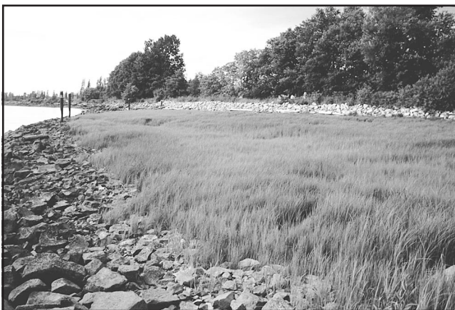
Figure 6. Constructed marsh at Deering Island, North Arm, looking downstream. Photo by M. Adams. GSC 2003-498
