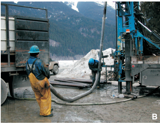
Figure 2. A) Drilling on Neil Vanloon's Farm (drillhole DHPV01; see Fig. 1). B) Extracting the core (drillhole DHPV11; see Fig. 1).
