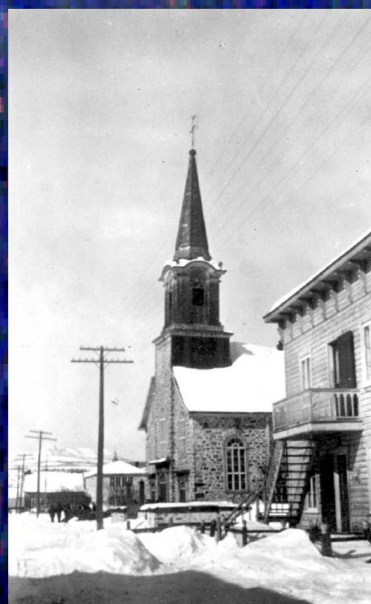
At Saint-Urbain, the church was heavily damaged and had to be demolished.
