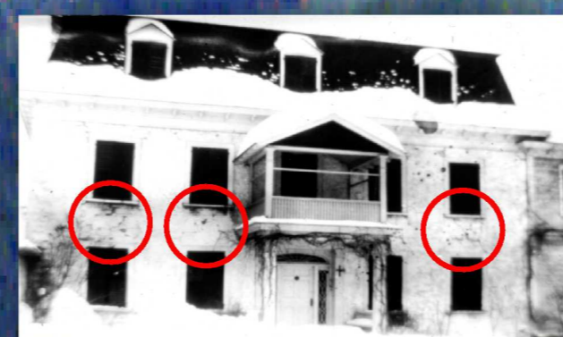
Several homes developed cracks in their masonry walls.
