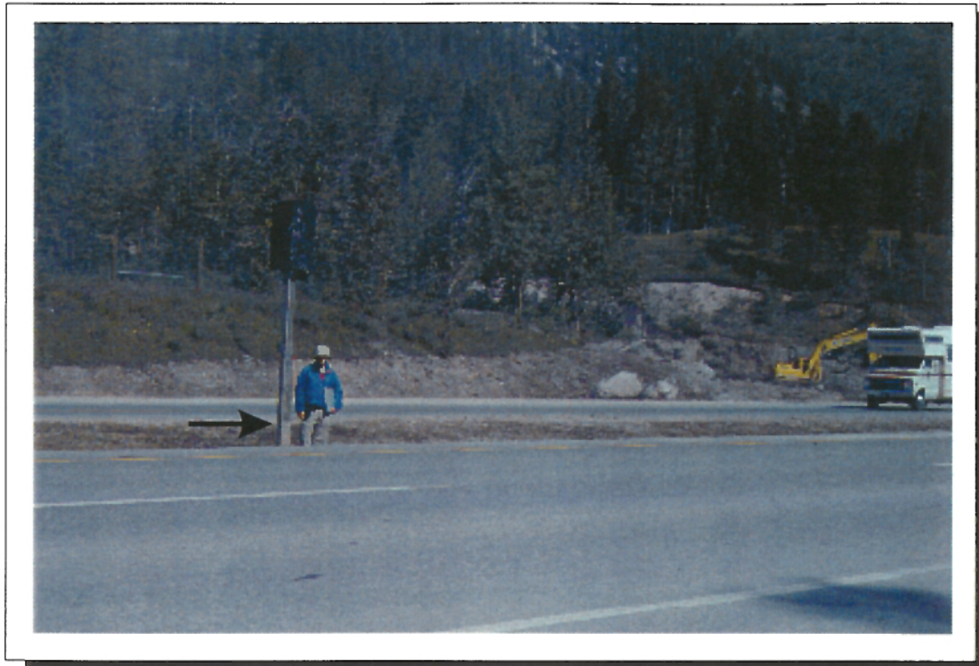
Figure 4.15 The debris flow overwhelmed the four-lane Trans Canada Highway. Three weeks after the debris flow all the debris was removed from the highway. Mud on a sign post indicates how thick the debris cover was over the highway, (about 30 cm, as pointed by the arrow). See Figure 4.3 for location of the photograph.
