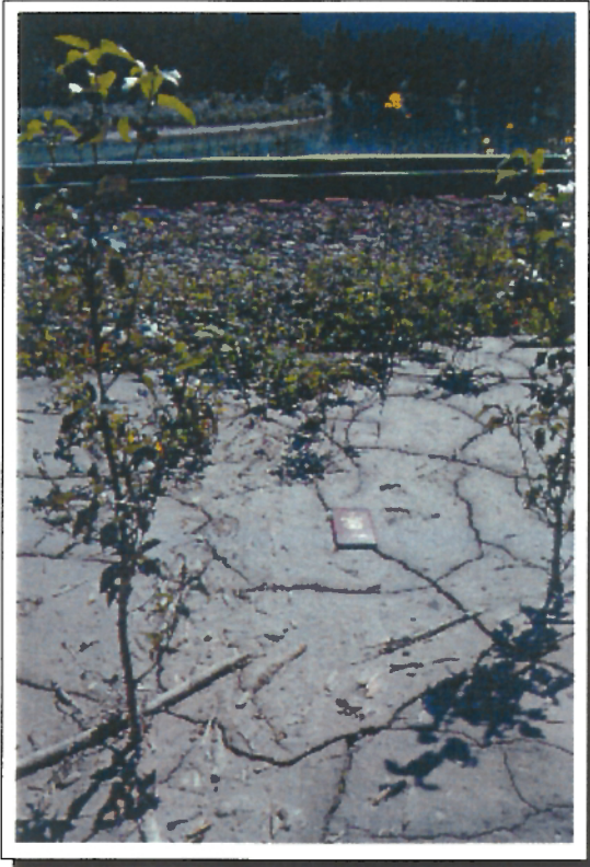
Figure 4.18 Photograph showing debris deposited beside the CP track. The average thickness of debris is 0.15 m, but can be thicker at some locations. Debris is essentially silty clay with gravel and organic matter. The field book gives the scale. See Figure 4.3 for location of the photograph.
