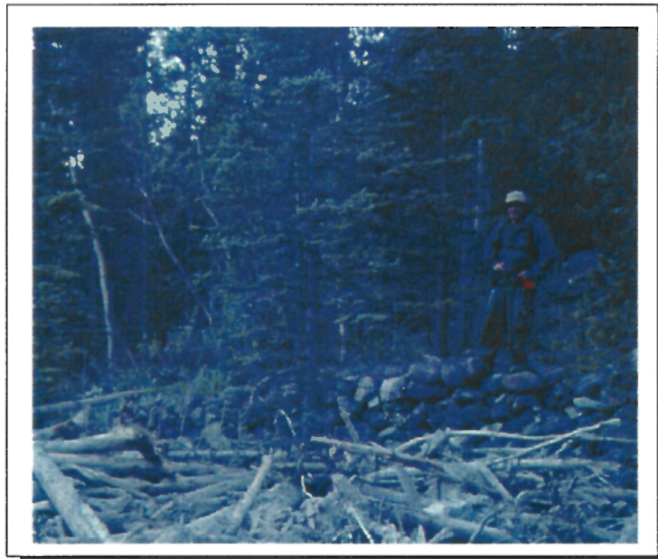
Figure 4.12 A section of a berm installed by Canadian Pacific Railway in the Fifties to deviate water flow through the middle of the fan. The berm was partially destroyed by the 1999 debris flow. Note the accumulation of wooden debris beside the berm. The berm is formed by man-made cemented pebbles and rounded boulders smaller than 30 cm. The berm was about 1 m high and 100 m long. A person gives the scale. See Figure 4.3 for location of the photograph.
