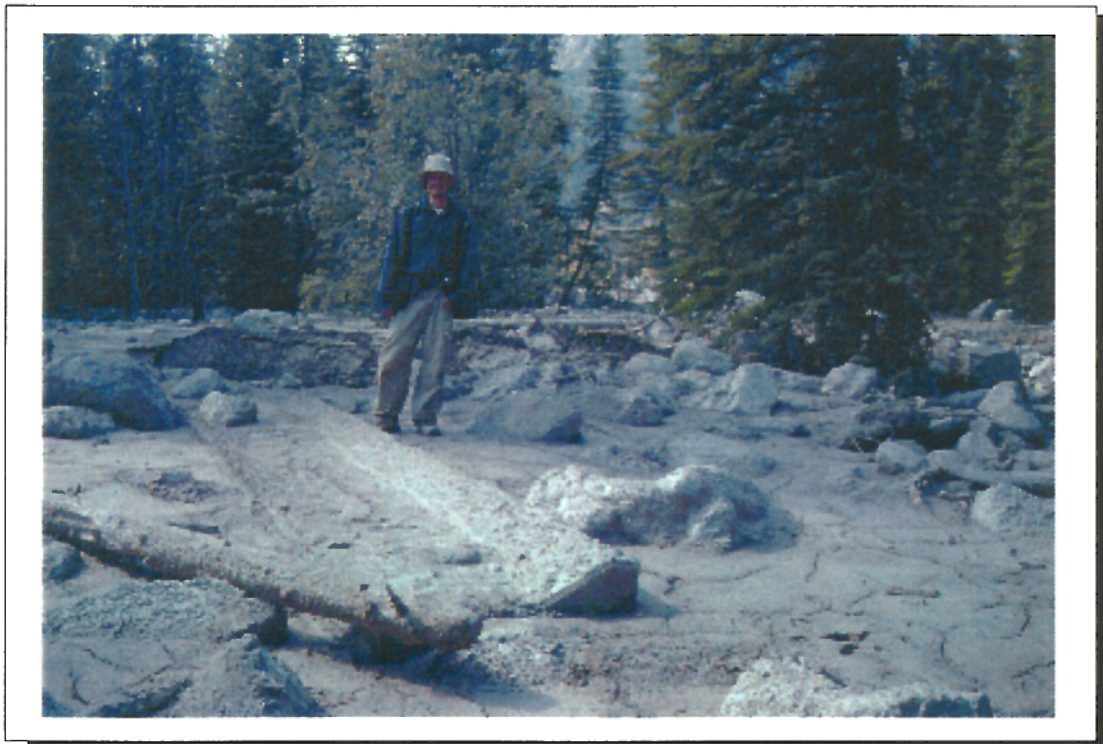
Figure 4.19 Photograph showing a section of a New Jersey concrete fence transported 200 m by the debris flow from its original location along the Trans-Canada Highway. Notice that coarser blocks are entirely covered by mud or fines (sample #5). See Figure 4.8 for grain size distribution. Figures 4.2 and 4.3 give respectively the location of the sample and the location of photograph.
