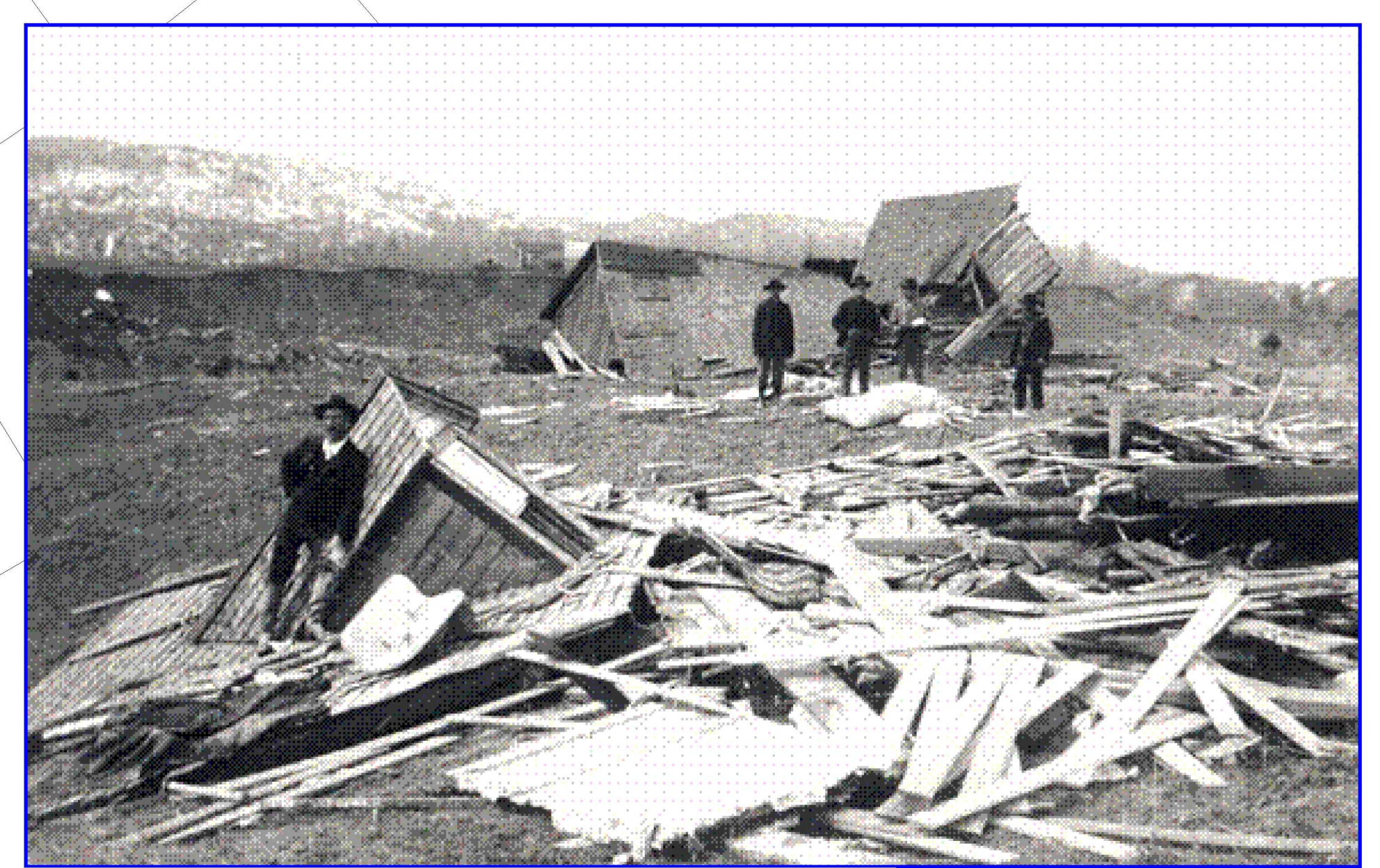
View of buildings destroyed in the village of Notre-Dame-de-la-Salette, Quebec by a wave generated by the 1908 landslide. The landslide in Leda Clay occurred on the right bank of the Lièvre River generating a wave which swept over the village on the left bank of the river, destroying 32 wooden buildings. 30 people were killed in the disaster (Disaster 15 in listing). Photograph courtesy of the Archives nationales du Québec.
