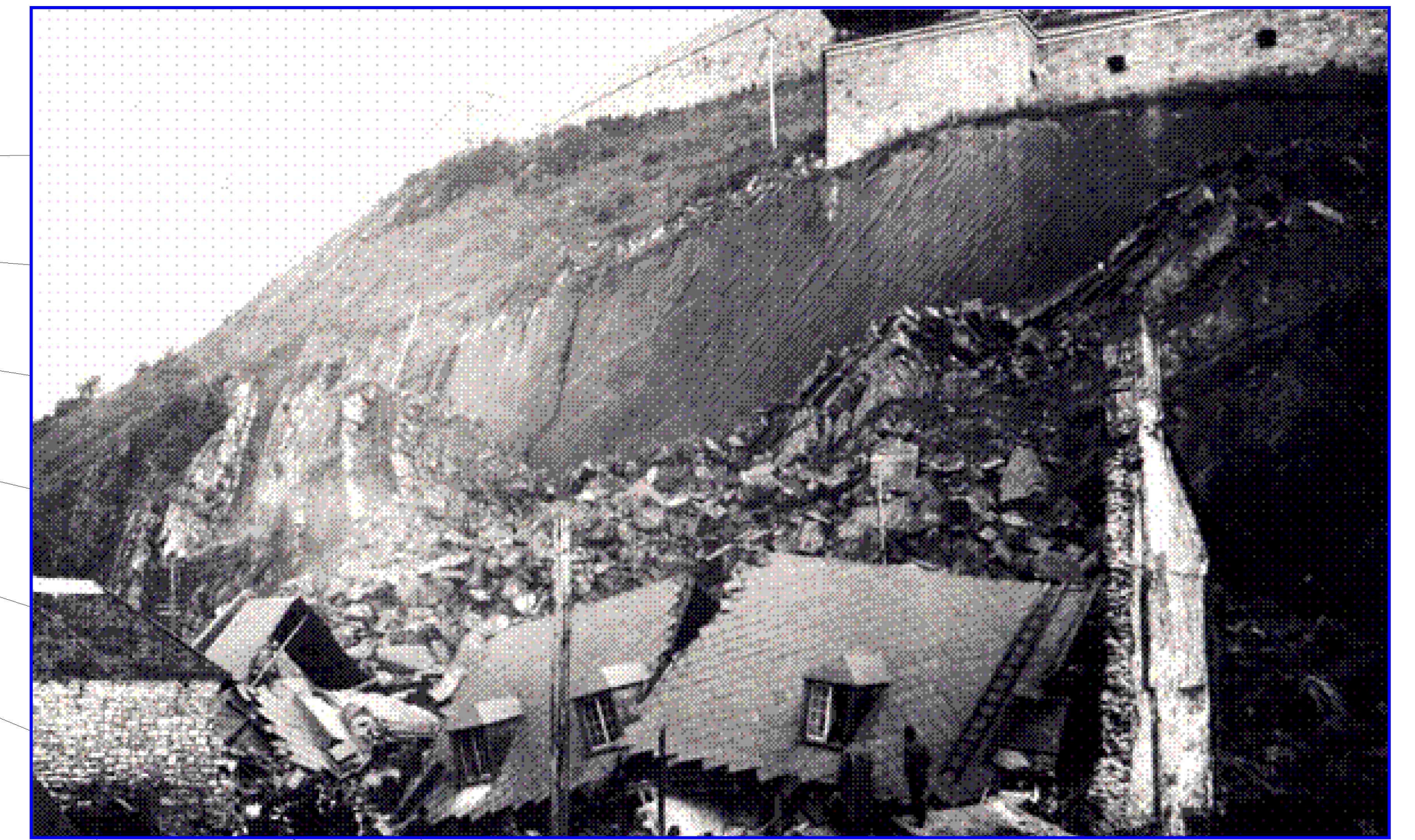
Houses destroyed by rockslide on Champlain Street, Quebec City, in September 1899. 50 people were killed in this landslide disaster (Disaster 5 in listing) which in eastern Canada's worst. The rockslide resulted from the failure of the slope behind the houses, just below the walls of the Citadel. Public Archives of Canada photograph.
