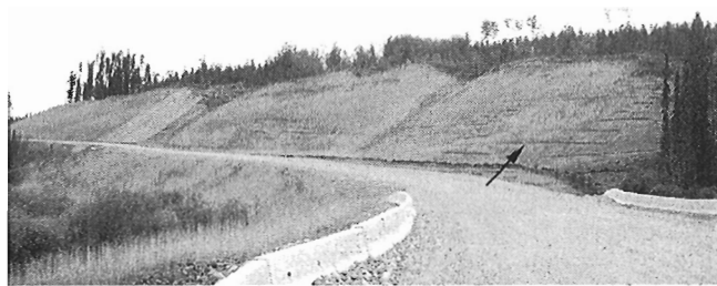
Figure 5. View of the road cut in glacial lake sediments at Big Bend Creek. Extensive working has been completed at this site to mitigate the instability of the sediments. Arrow points at willow wattles.
