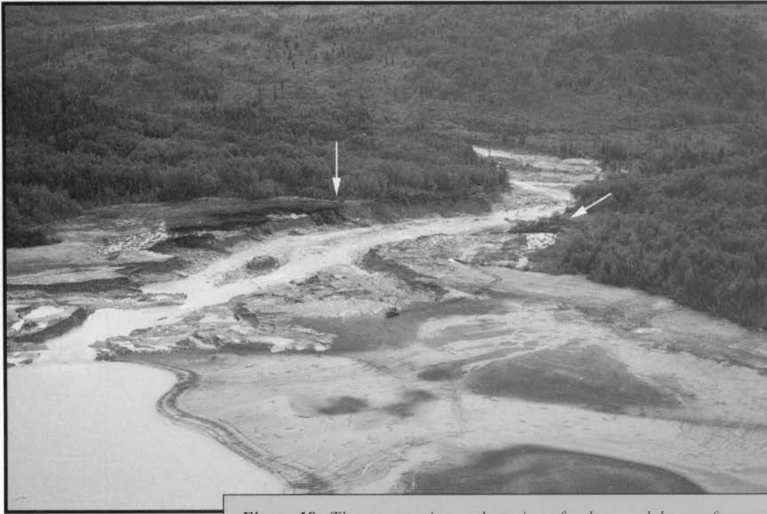
Figure 19. The overtopping and erosion of a dam or dyke can form a breach that progressively enlarges over time, increasing the outflow of water. The rate of erosion of the breach depends on a number of factors including the shape, height, width, length, and composition of the dam or dyke and the volume of impounded water available for drainage. Outflow will begin to decrease when the supply of water wanes as the reservoir level falls or outlet erosion slows. Breaching of a dam or dyke can result in the catastrophic release of water the discharge of which is generally directly proportional to the volume of water stored in the reservoir (see Costa, 1988).
