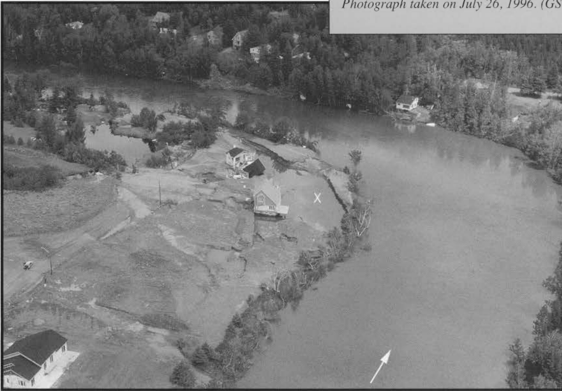
Figure 6. Localized floodplain erosion can occur where turbulent eddies and separated flow develop to the lee of objects (e.g. trees, fences, and buildings) located along the riverbank or on the floodplain surface (see for example Miller and Parkinson, 1993). In this photograph, a large, elongated scour hole ('x') occurs on the floodplain along the Chicoutimi River. It was likely formed by turbulence generated to the lee of a row of small trees growing on the edge of the riverbank. Note the two houses damaged by inundation by the floodwaters and undermining by erosion of the scour hole. The arrow indicates the direction of river flow. Photograph taken on July 26, 1996. (GSC 1997-42V)
