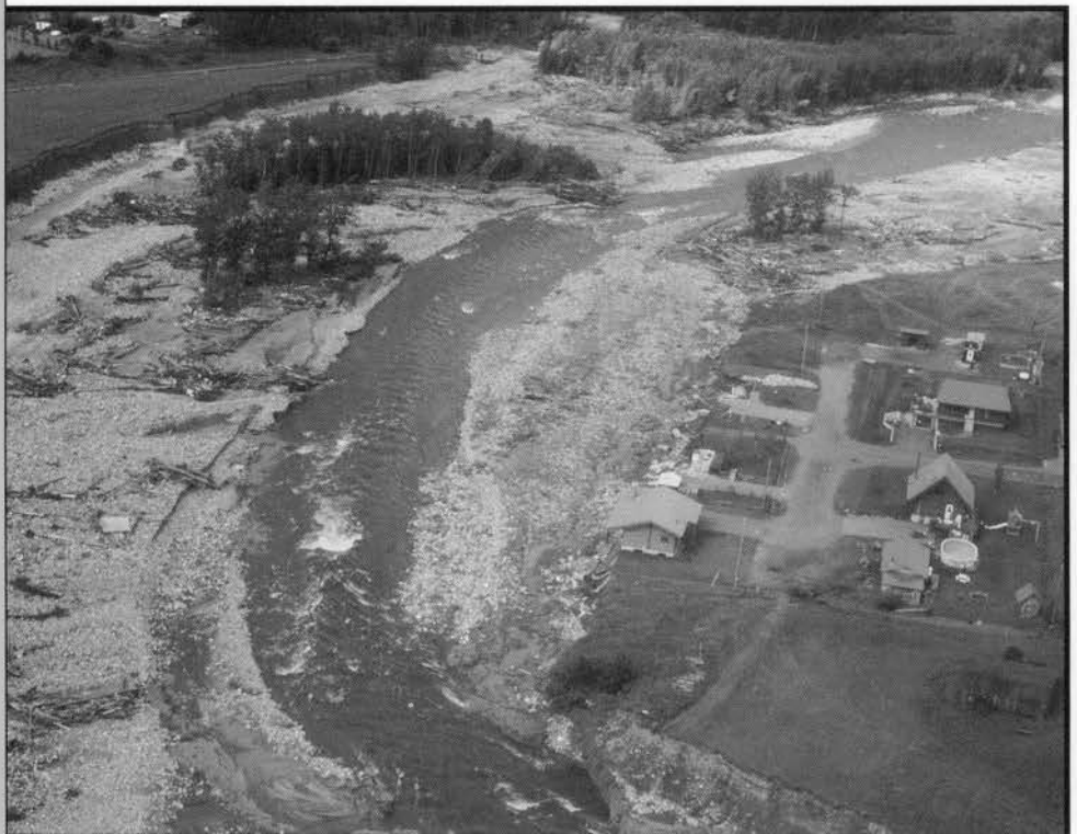
Figure 9. Inherent to the large-scale widening of a river channel during a major flood is the lateral erosion of floodplain and terrace deposits along the river margins. The extensive widening that occurred along both the lower à Mars River and the Ha! Ha! River during the flood was caused, in part, by the lateral erosion of terrace deposits along floodplain margins. Some houses located near the edge of the eroding terraces were damaged or destroyed by undermining associated with bank erosion. At this site along the à Mars River, one house overhangs the riverbank and several adjacent houses have been destroyed. The loss of or damage to these houses is particularly notable as they are located above the level of flooding. Photograph taken on July 27, 1996. (GSC 1997-42DD)
