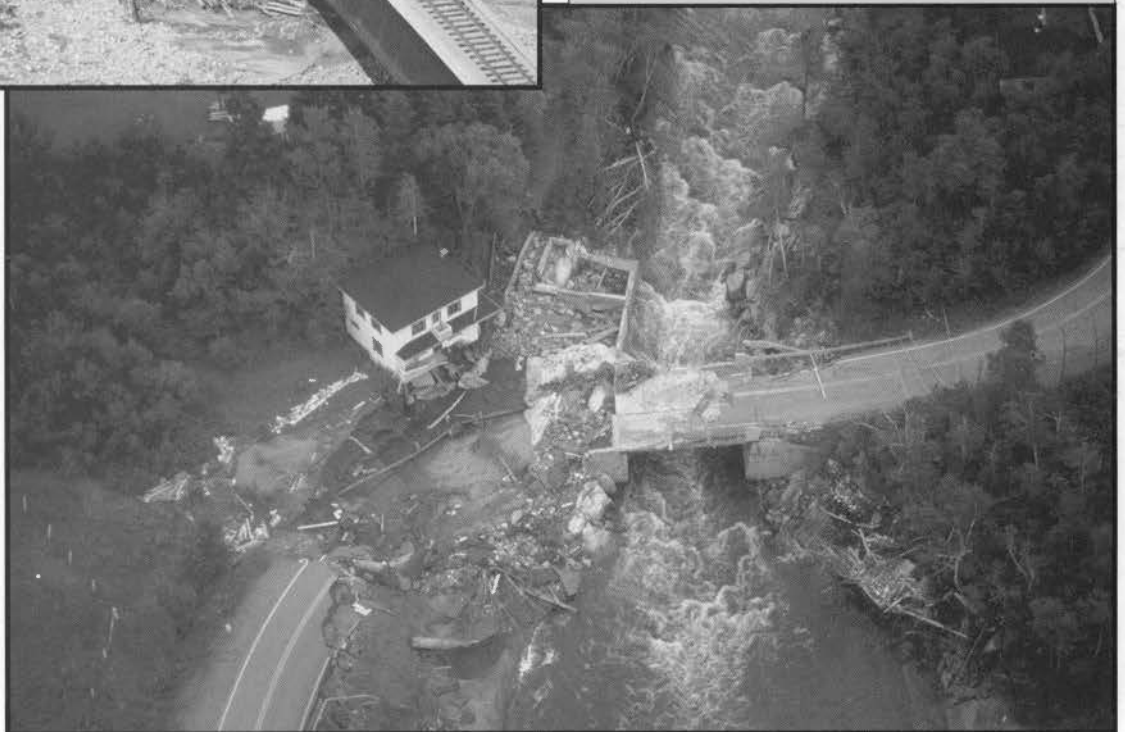
Figure 13. The à Martel Falls along the du Moulin River provide another example of damage at a bridge site. Here, floodwaters spilled over a bridge that constricts a narrow reach of the river. The overflow washed out the road and severely damaged two houses next to the river. Although the bridge was damaged, its basic structure remains intact. Photograph taken on July 27, 1996. (GSC 1997-42WW)
