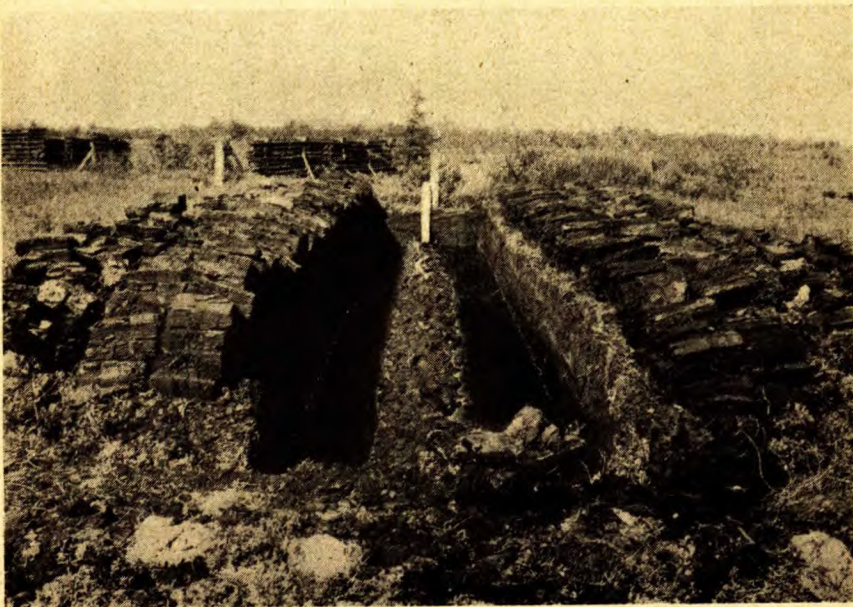
B. Digging a ditch, with peat sods piled at sides.
