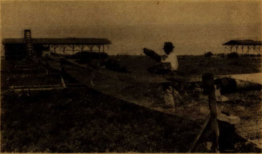
A. Belt conveyer taking peat to field storage sheds.
