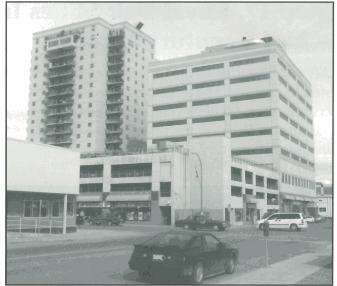
Figure 54. Stop 15 – The Centre Square Mall, built on reinforced piles secured to bedrock. GSC 1998-006 X
