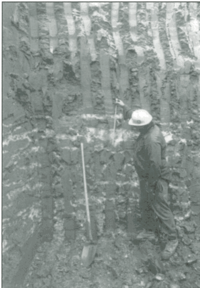
Figure 68. Excavations along Franklin Avenue in 1990 revealed a substantial amount of ice in the form of ice lenses. The man in the photo is measuring ice lenses, which look like white layers in the soil. (Photo by Walter Orr)
