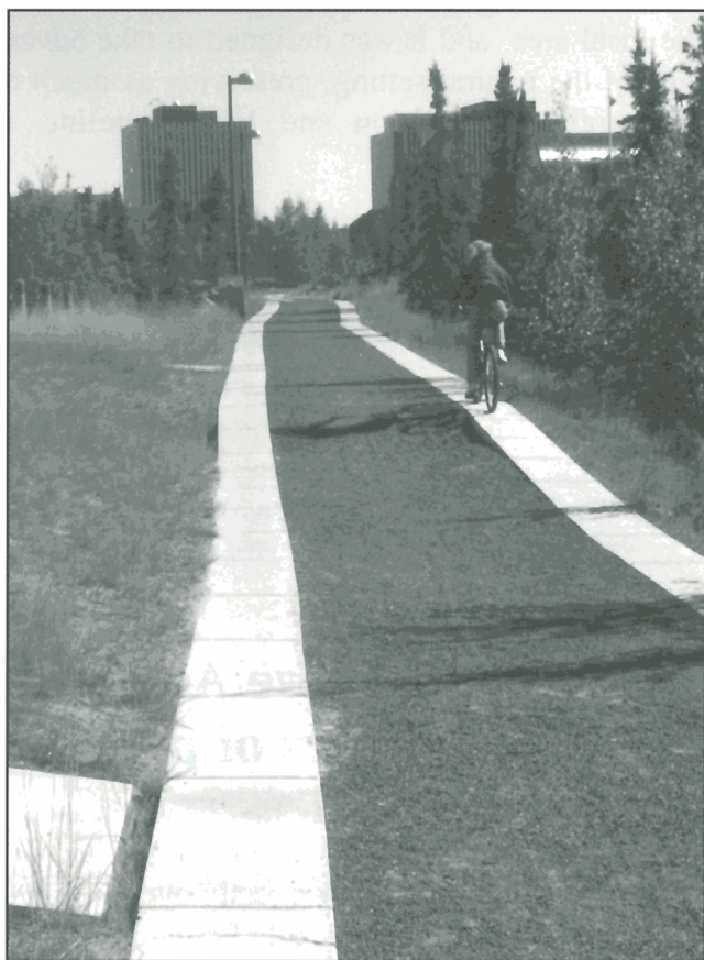
Figure 37. Stop 4 – Settlement of the walking trail between the Legislative Assembly and Prince of Wales Heritage Centre, caused by thawing of the underlying permafrost. GSC 1998-006 N
