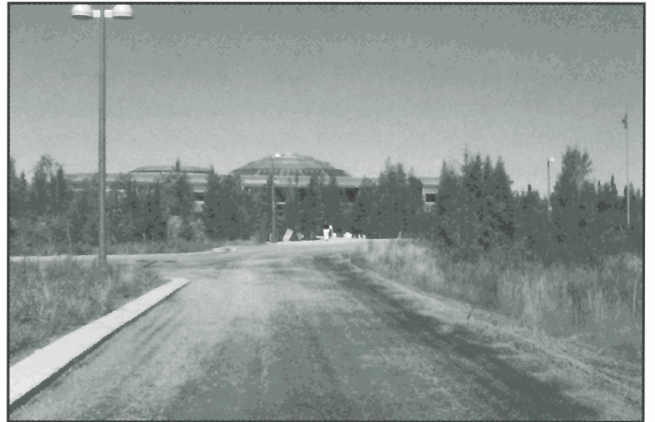
Figure 36. Stops 2 and 3 – The Legislative Assembly. Permafrost exists beneath the gravel road in front of the Legislative Assembly building. The roadway was paved in 1997, with precautions taken to preserve the permafrost. GSC 1998-006 M
