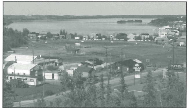
Figure 71. View across Back Bay with Fritz Theil Park (Stop 28) in centre. GSC 1998-006 KK
