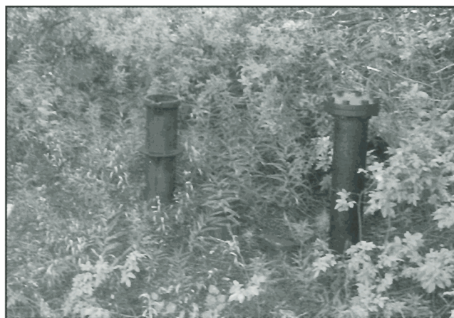
Figure 72. The old sewage line running to Niven Lake is still visible in a few places. GSC 1998-006 LL
