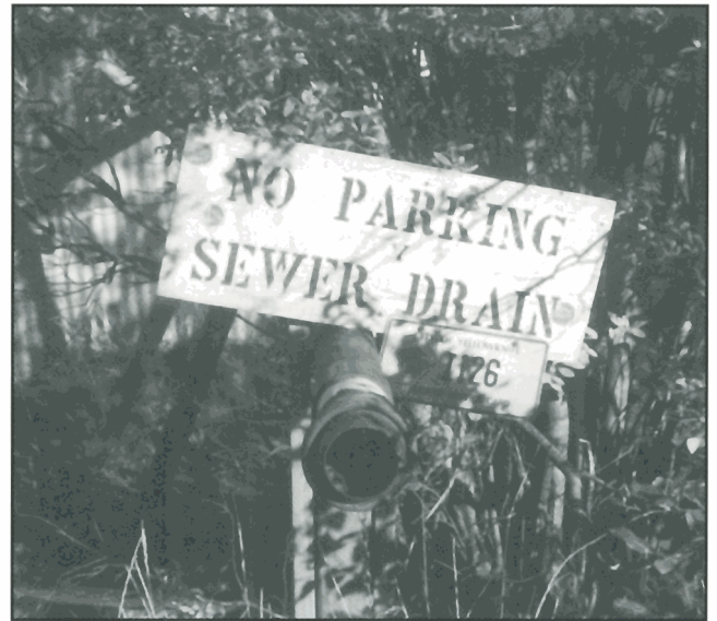
Figure 66. Residents of the Old Town area have sewage trucked out because of the difficulty of placing sewer lines in the rocky terrain. Water is piped into homes in the summer, and trucked in in the winter. GSC 1998-006 HH
