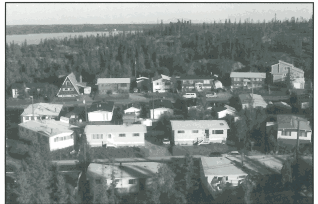
Figure 61. Stop 22 – School Draw subdivision. Because of settling caused by the thawing of permafrost, most of the houses in School Draw had to be removed from their foundations and the foundations rebuilt using piles anchored to bedrock. GSC 1998-006 DD
