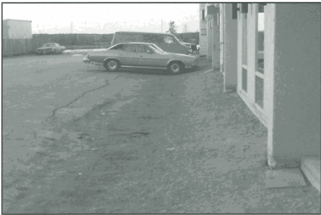
Figure 44. Settlement beside the Bowling Green building on 49 Street. (Photo by Larry Aspler, October 1977)
