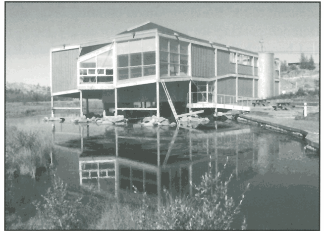
Figure 43. Stop 8 – Part of the Visitors Centre rests on piles. GSC 1998-006 S
