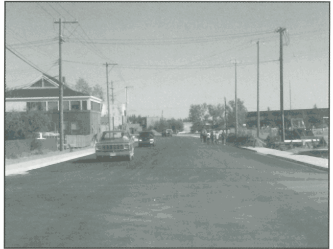
Figure 58. Stop 18 – The corner of 49 Street and 52 Avenue. The problem soils beneath 52 Avenue were removed and the road was repaved in the summer of 1997. How does it look now? GSC 1998-006 BB
