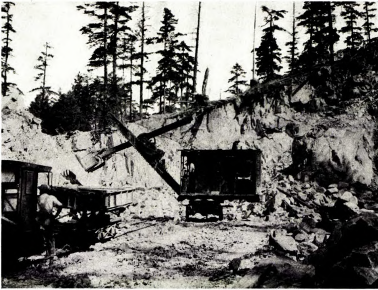
A. Part of quarry of British Columbia Cement Company, Ltd., Blubber Bay, Texada island, B.C.
