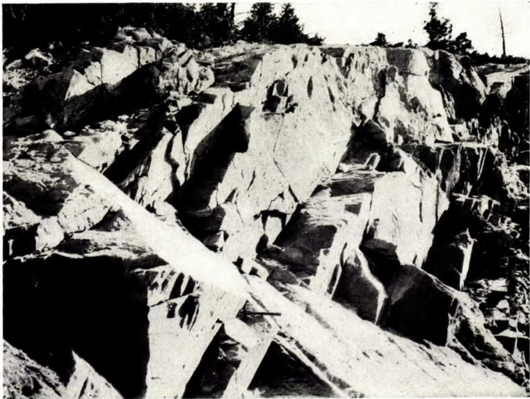
B. Heavily bedded Devono-Carboniferous limestone with irregular jointing, East quarry of Summit Lime Works, Ltd., Crowsnest pass, Alta.
