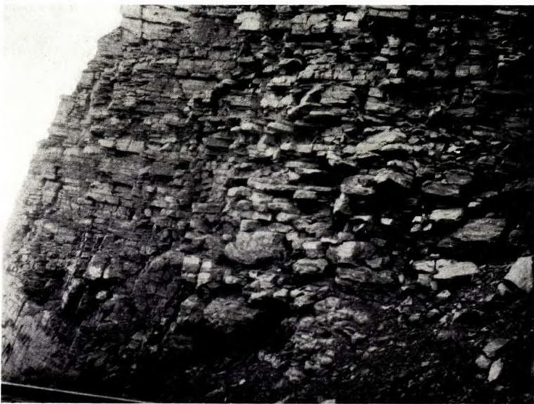
B. Thinly bedded, Devonian-Carboniferous limestone in railway cutting at Mile 148, Nordegg, Alta.
