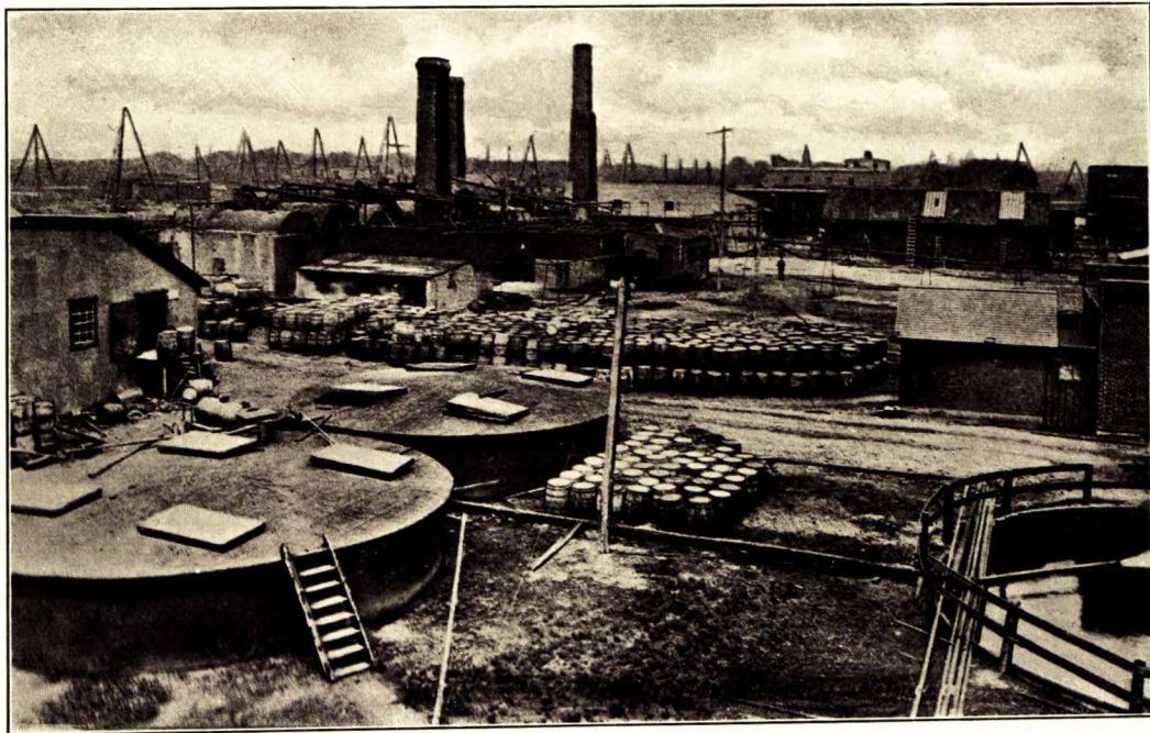
Canadian oil refinery, Petrolia, Ont.
