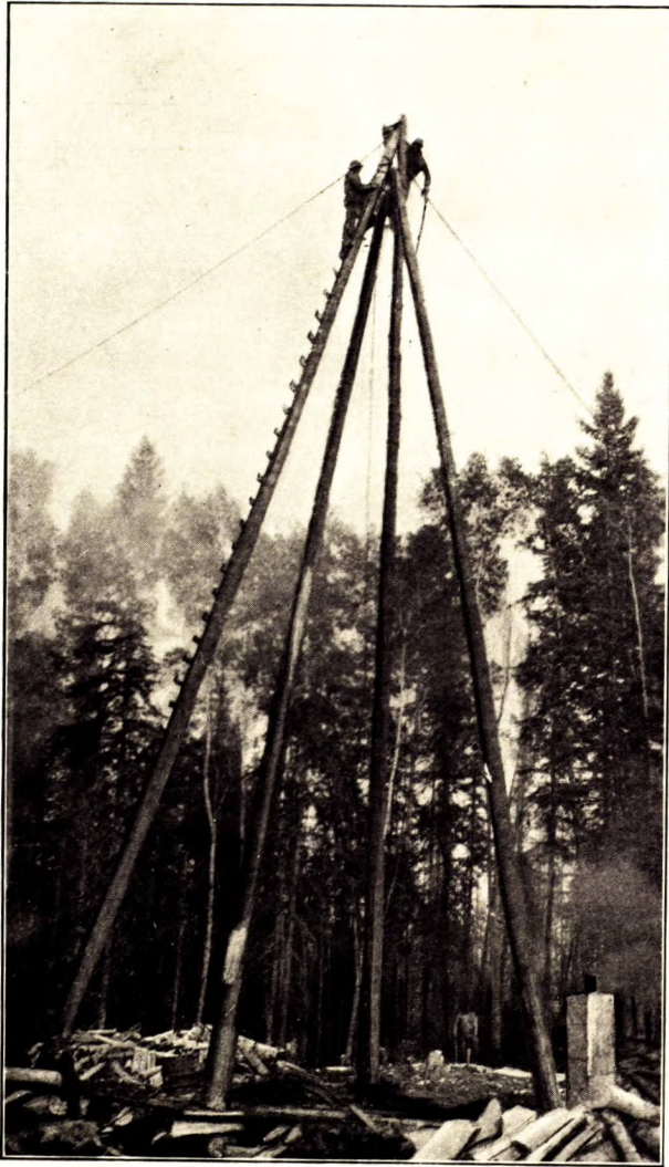
Derrick at No. 2 well in course of erection, Athabaska Oils, Ltd., 9 miles below Fort McKay, Alberta.
