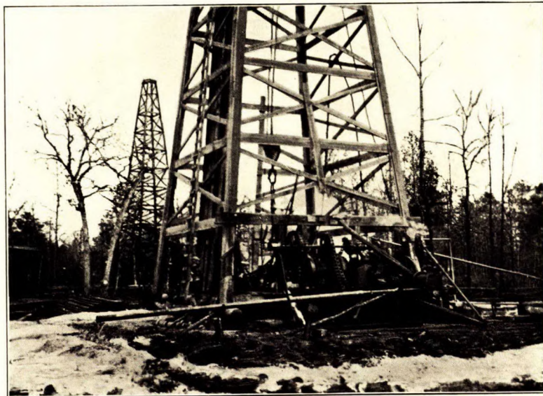
Rotary method of drilling, Caddo field, La., U.S.A.
