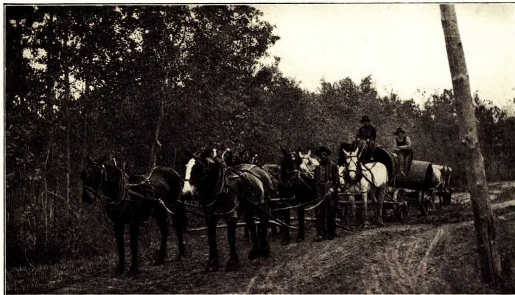
Hauling boiler from Edmonton to Athabaska, Alberta, 1911.
