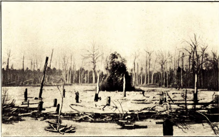
Blown out gas well, Caddo field, Oil City, La., U.S.A. (The position occupied by the columns of water is the site of a well which was blown out.)
