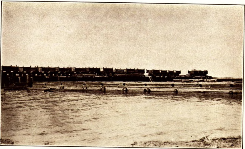
B. Loading pier and train of cars, Windsor Gypsum Company, Windsor, N.S.
