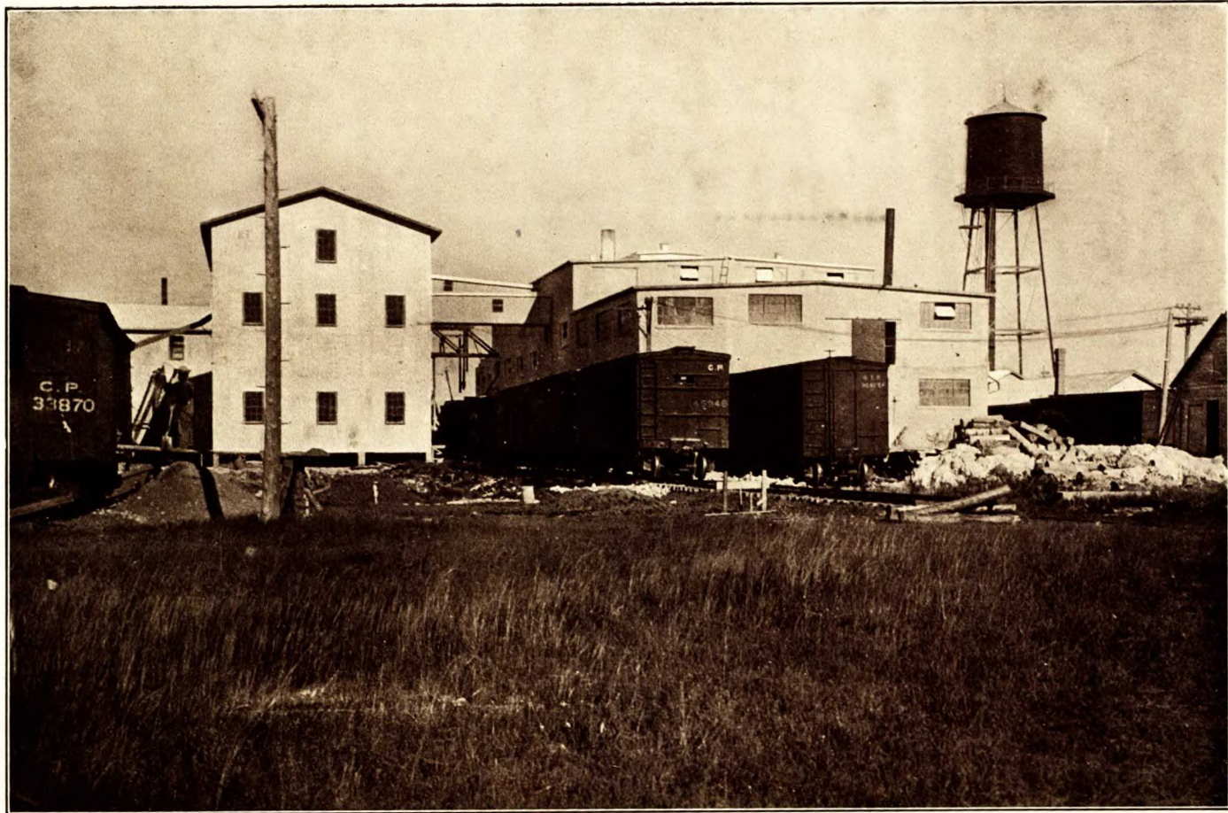
Mill buildings of the Manitoba Gypsum Company, Winnipeg, Man.
