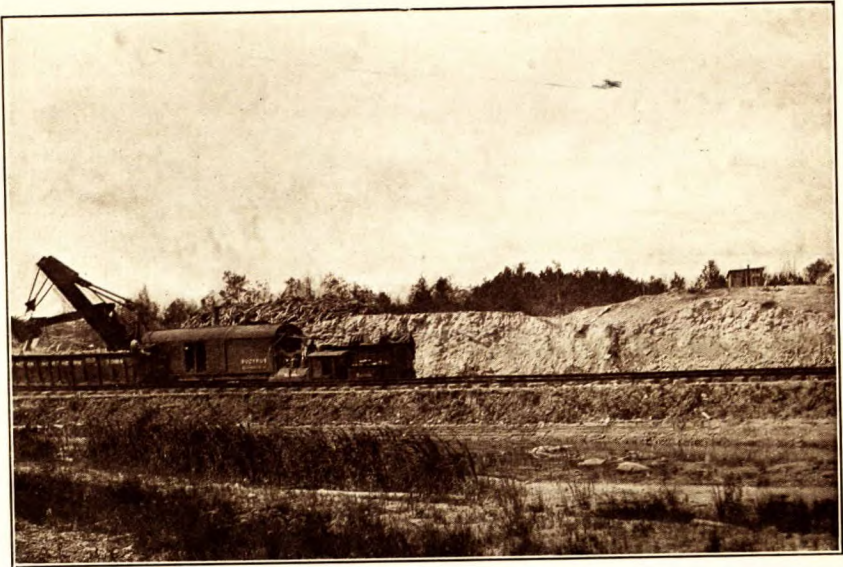
A. West face of quarry, with steam shovel, Manitoba Gypsum Company, Gypsumville, Man.
