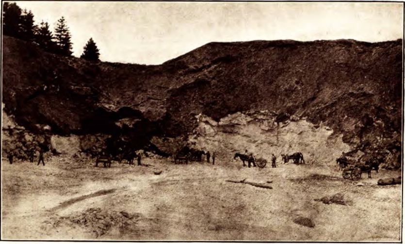
A. Wentworth Gypsum Company's quarry, looking west from loading platform. (Note thickness of overburden.)
