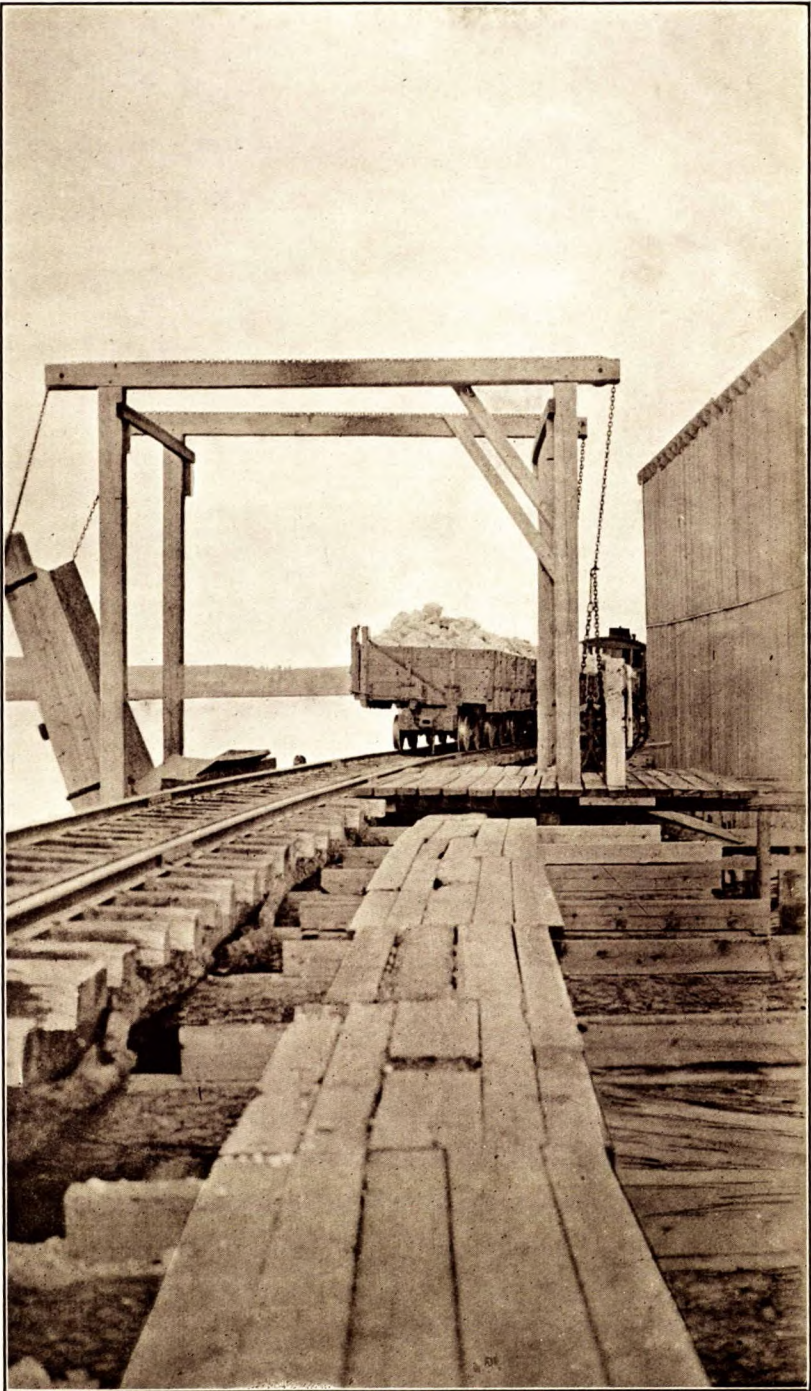
Shipping pier and loading device, Wentworth Gypsum Company.
