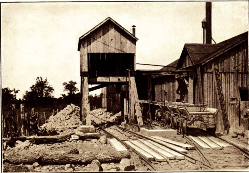
B. Hoisting apparatus and cars, Crown Gypsum Company, York, Ont.
