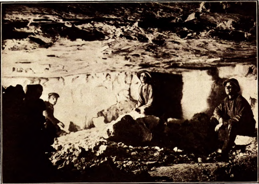
B. View underground in mine of Crown Gypsum Company, York, Ont., showing width of bed being worked.
