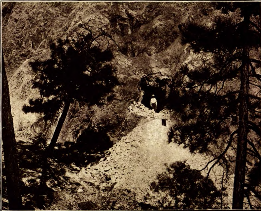
B. Closer view of tunnel, Spatsum deposits, Spatsum, B.C. Material on dump, principally altered limestone with occasional blocks of gypsum.
