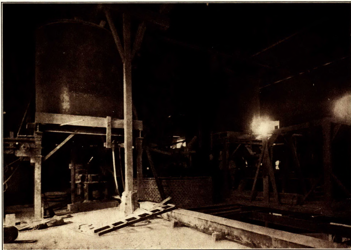
Interior view of mill of Alabastine Company, Caledonia, Ont., showing steel storage bins above kettle, and one kettle in place.
