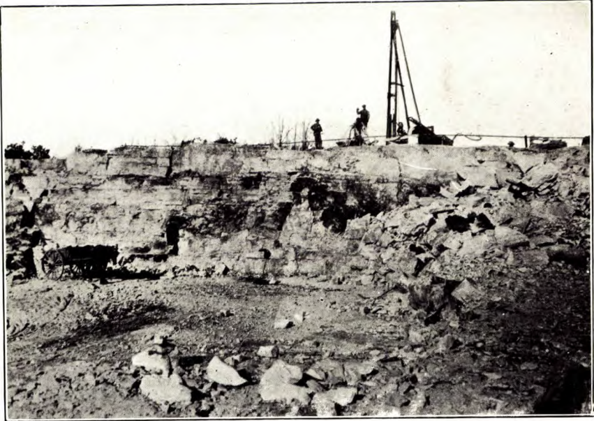
A. Quarry of Silico Ltd., at St. Canute, Que.
