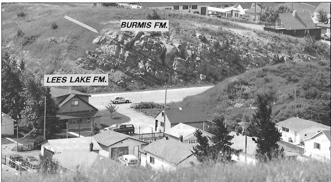
Figure 3. Uppermost Alberta Group formations exposed along Highway 3 at Coleman. View toward the southwest from the Forestry Trunk Road.
