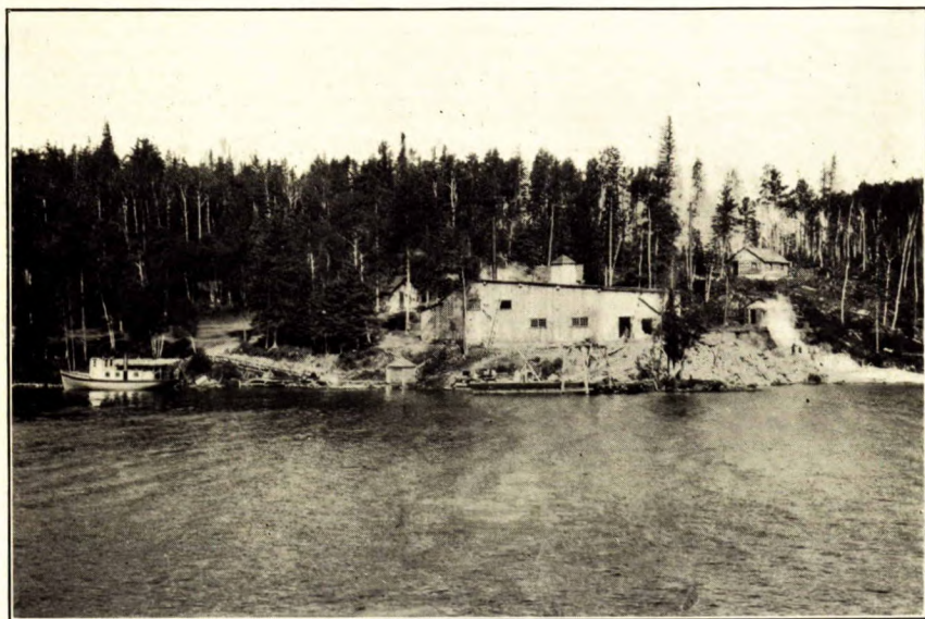
A. General view of soapstone quarry of Grace Mining Company, on Eagle lake, Ontario. Sawing-shed is shown at left of pit.
