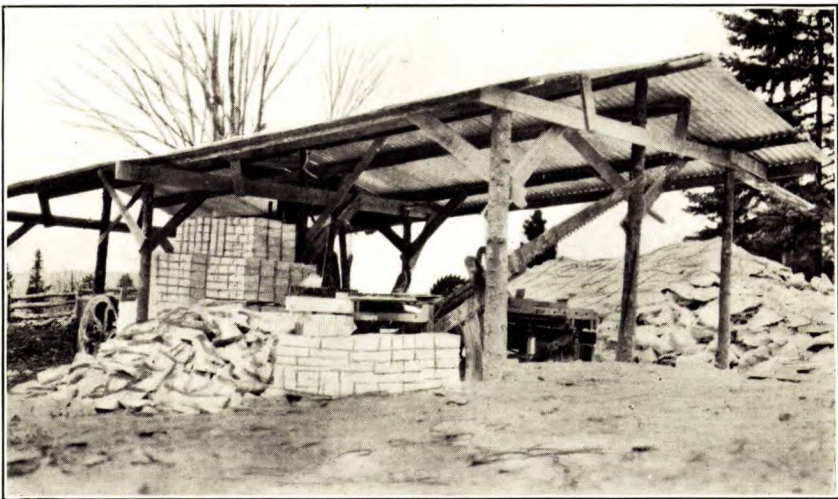
B. Type of portable, sawing equipment employed by Robertsonville Soapstone Company, Leeds and Thetford townships, Quebec.
