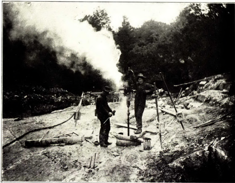
Rock Drill mounted on Quarry Bar.
