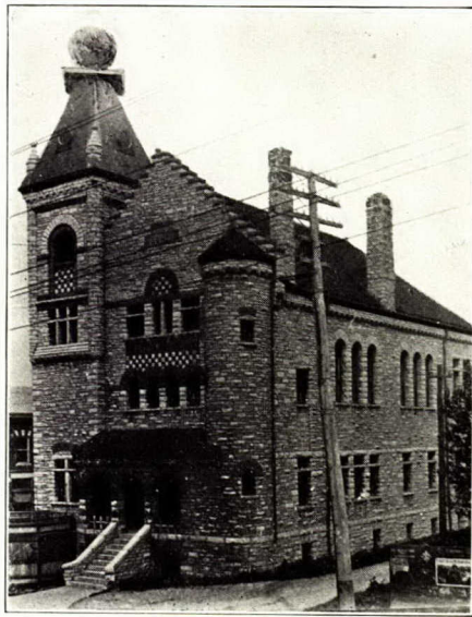
Onondaga Limestone. Municipal Buildings, St. Mary's, Ont.
