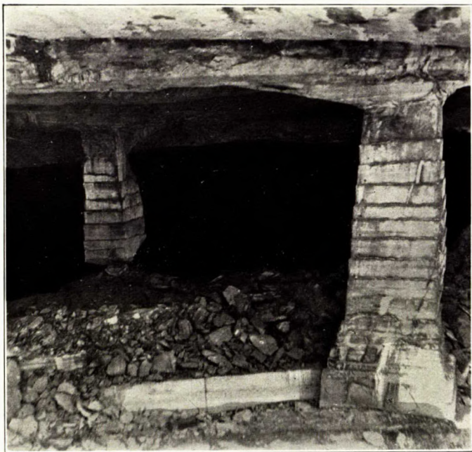
Marble Pillars left to support roof in tunnelling, West Rutland, Vt.
