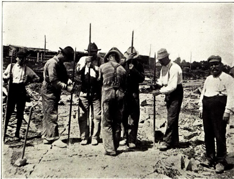
Drilling Plug Holes with Ball Drills, Longford Quarries.
