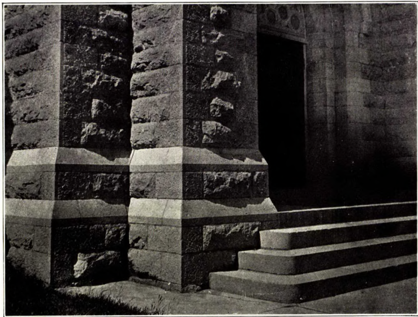
Crookston Limestone. Abutments, Roman Catholic Church, Belleville, Ont.
