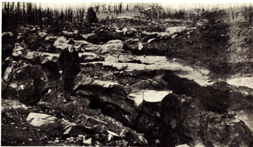
A. East part of vein-stripping, about 75 feet in length, showing tongues of vein separated by narrow horses of gneiss and pegmatite. (Photograph taken November, 1929.)
