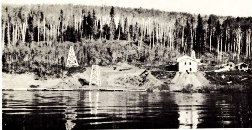
A. General view showing newly opened quarry on left, and separation plant building on right.
