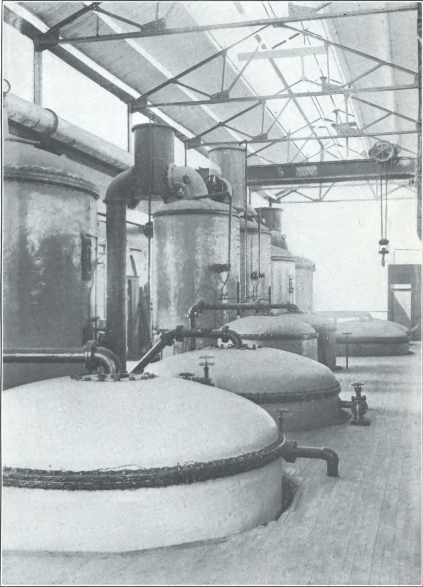
Vacuum evaporators (Scott type) for the concentration of caustic soda solutions. Canadian Industries, Limited, Sandwich, Ontario.
