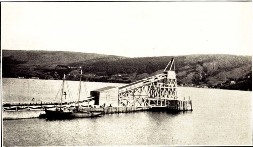
B. Conveying-belt and shipping pier, Ingonish Gypsum Company, Ingonish, Victoria county, Nova Scotia.
