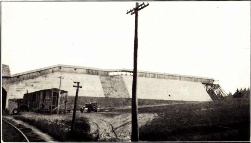
B. Storage sheds of the Atlantic Gypsum Products Company, at shipping pier, Walton, Hants county, Nova Scotia.
