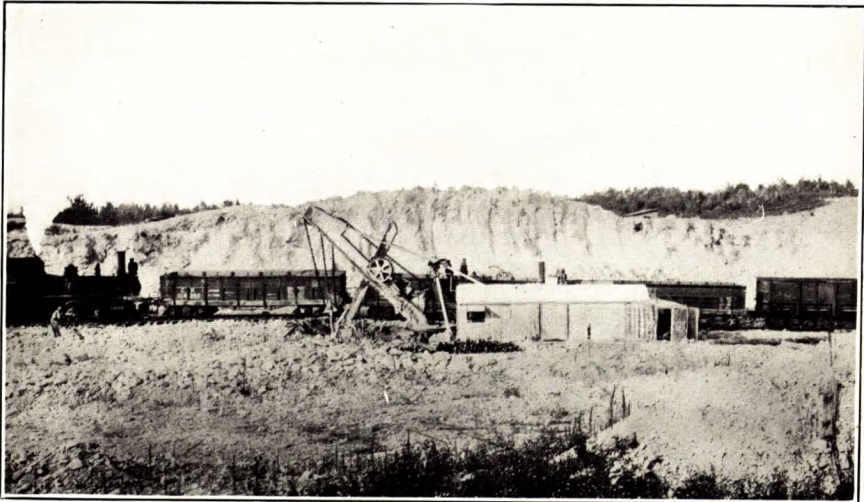
B. Steam shovel at work loading railway cars in the quarry of the Gypsum, Lime and Alabastine, Canada, Ltd., Gypsumville, Manitoba.
