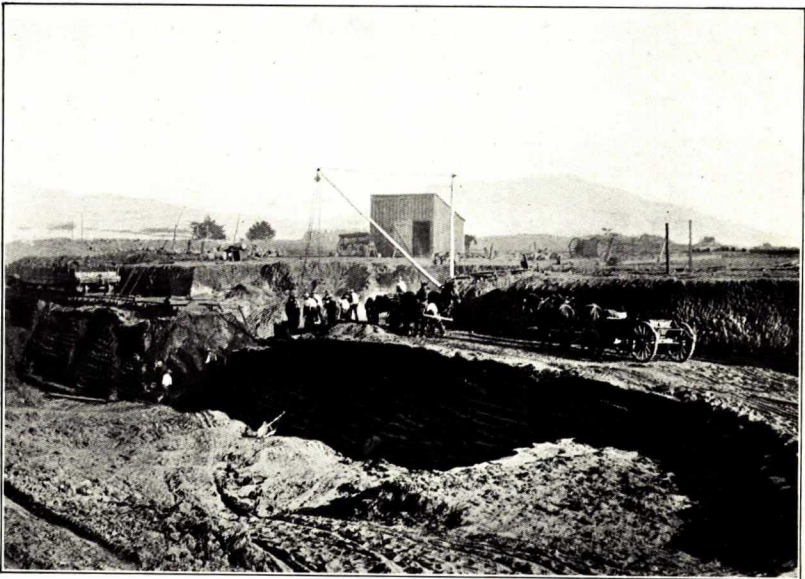
Quarry operated by A. Sattler, near Carpenteria, Cal., showing method of cutting down the asphalt in steps. The material is loaded into carts or railway cars, depending on where it is to be used.
