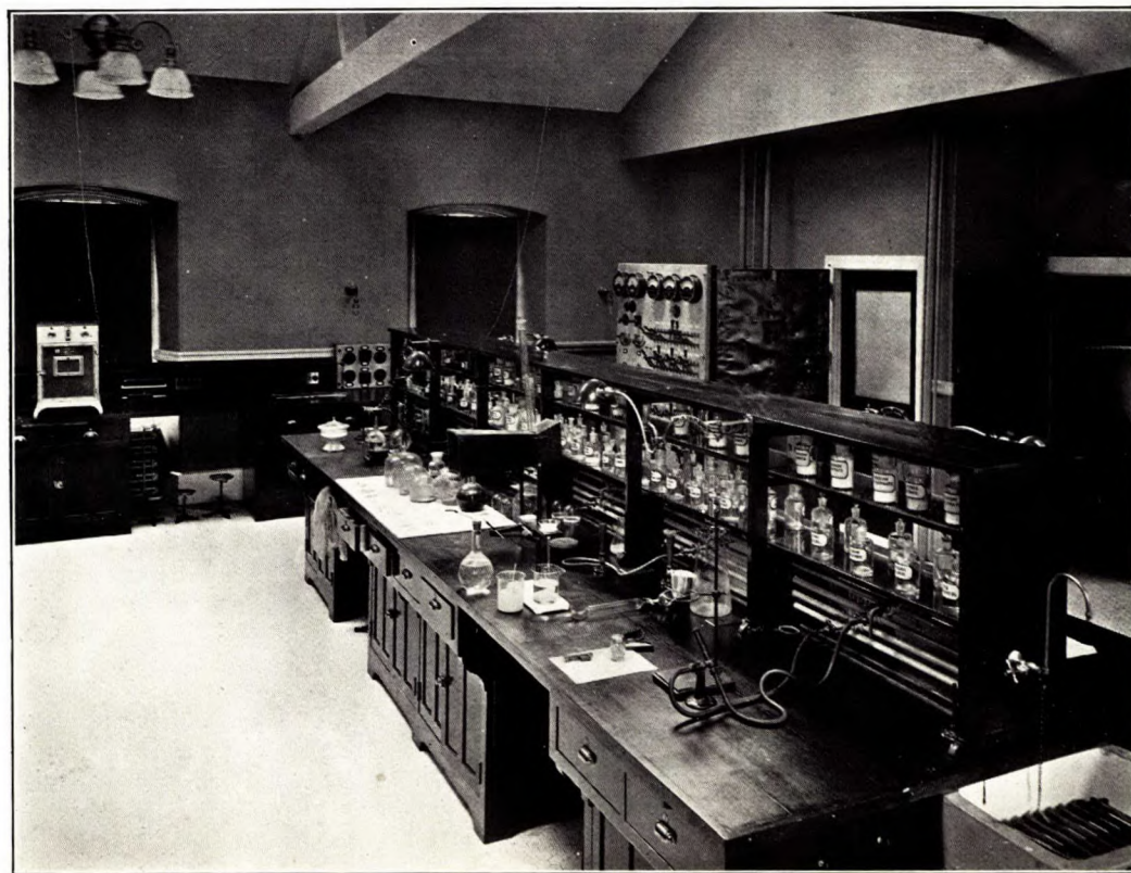
Main chemical laboratory: work table and electrical equipment.
