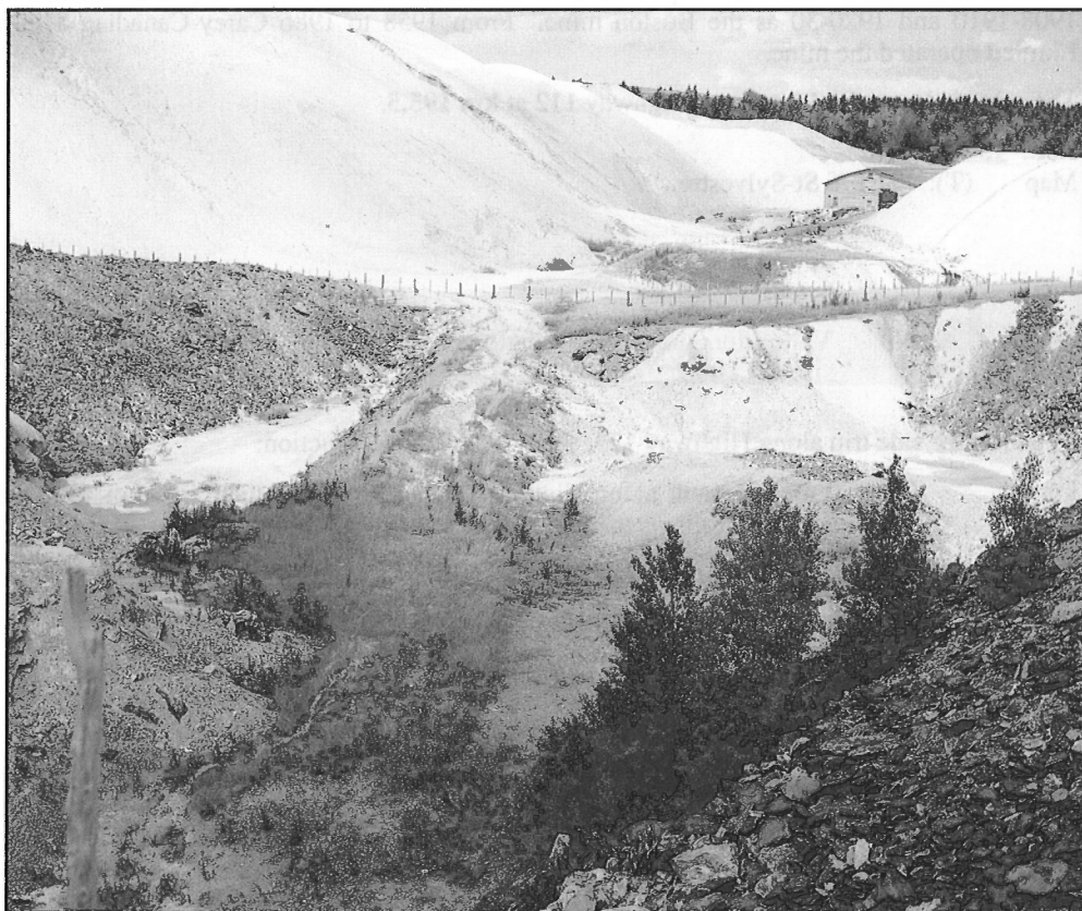
Plate XIII. East Broughton (Fraser) mine, 1965. White tailing dumps similar to those in the background are typical of the asbestos mining region. (GSC 138719)
