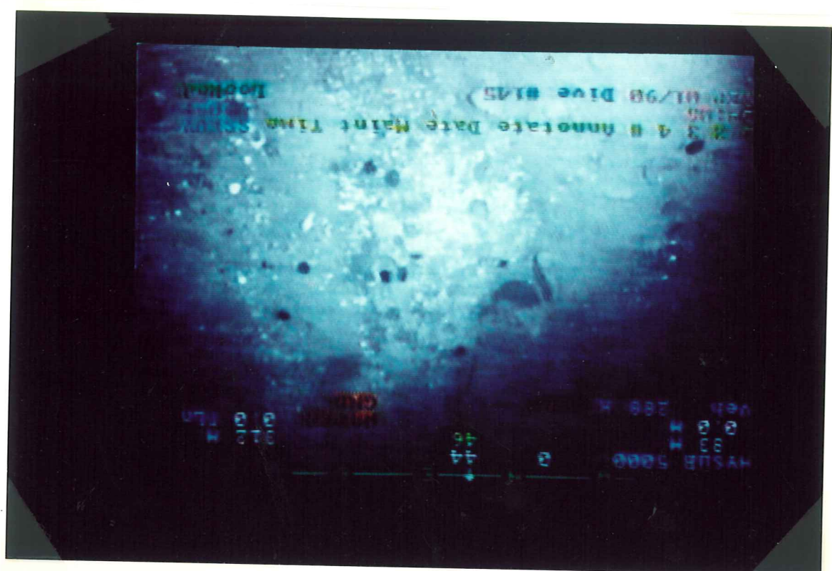
Fig 6I Sediment infill on glory hole floor. The large photo was taken directly from a high resolution monitor, the smaller photo was taken from a commercially processed image.
