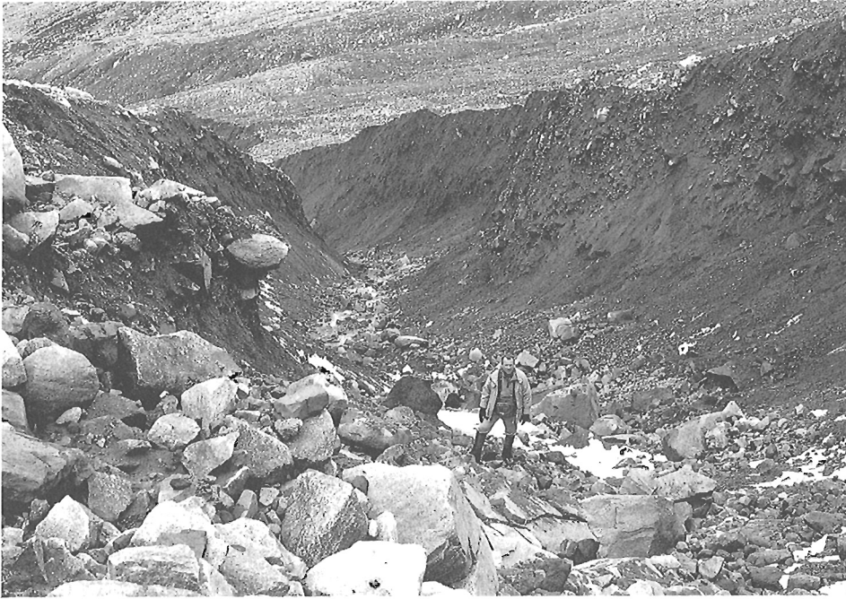
Figure 4. Trench on the outer flank of the moraine; view to the southwest. Person in foreground for scale.
