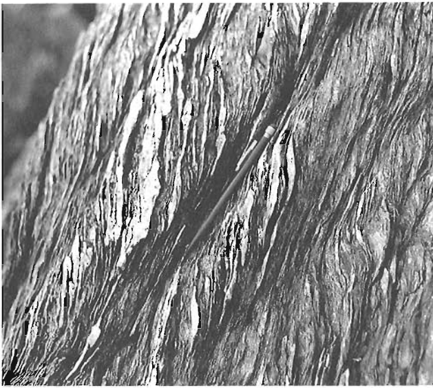
Figure 7. Section view of shear bands in sericite-chlorite schists of the coastal section, showing evidence of a reverse movement.
