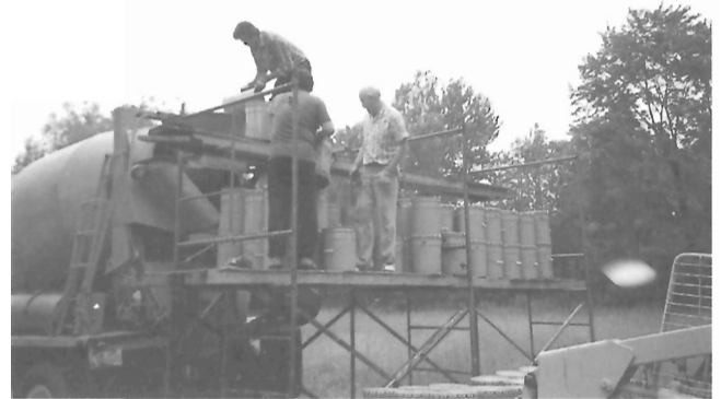
Figure 7. Phosphate slag being loaded into the cement truck. GSC 1991-130
