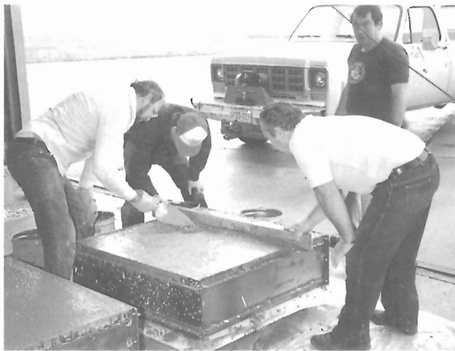
Figure 6. The metal forms used for pad construction. GSC 1991-124
