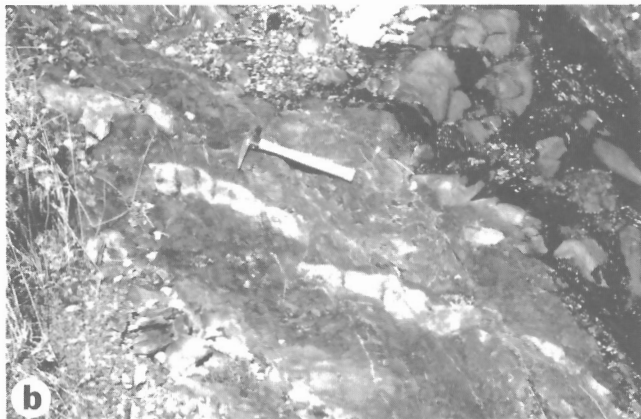
Figure 2. A. Outcrop of Eocene/Oligocene shale above Gosset Bay showing fissility ( S_1 ) shallowly inclined to bedding ( S_0 ). B. Minor faults in concretionary shale showing approximately 10 cm right-lateral offset. Fault surfaces are oriented approximately north-south.
