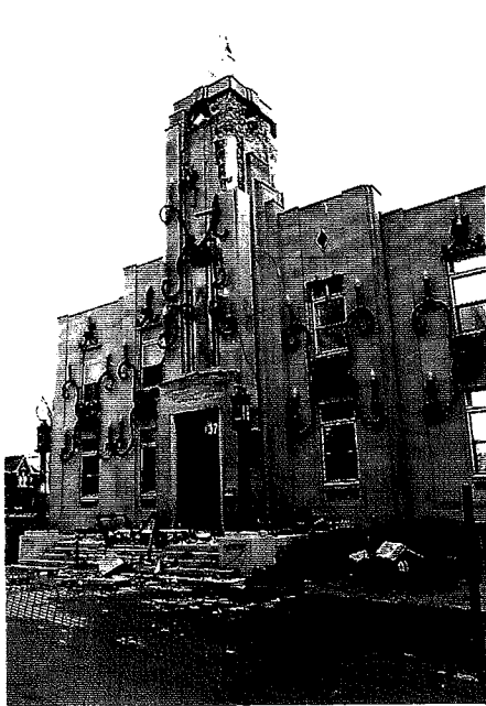
Debris from fallen masonry blocks in Dominique Racine Secondary School, Chicoutimi
