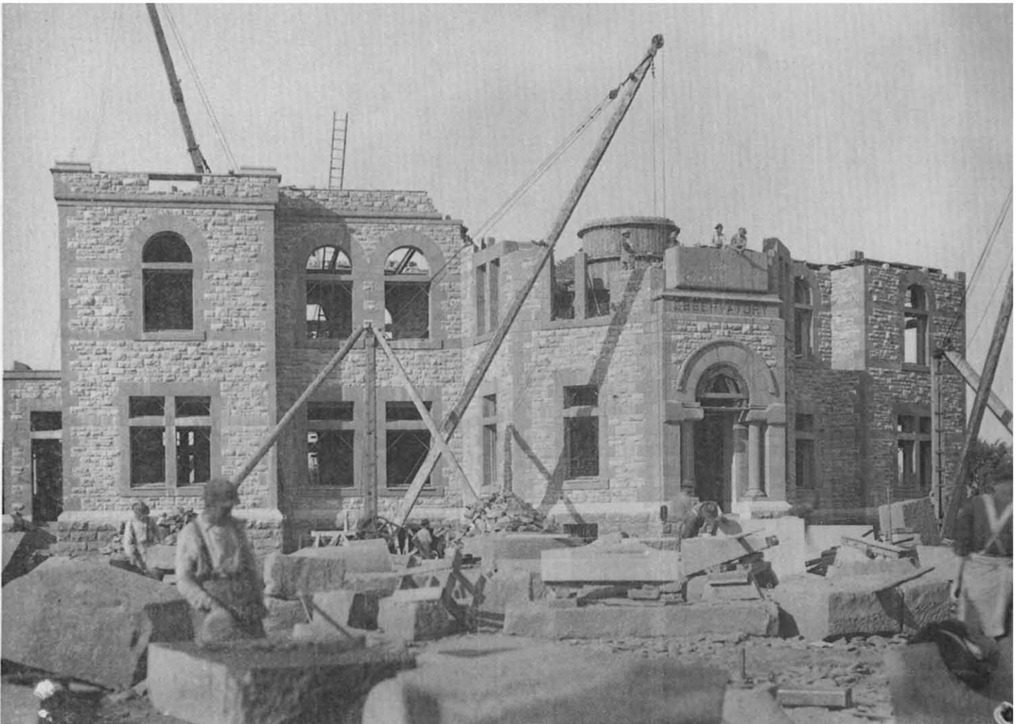
(Above and facing page) Construction of the Observatory.
