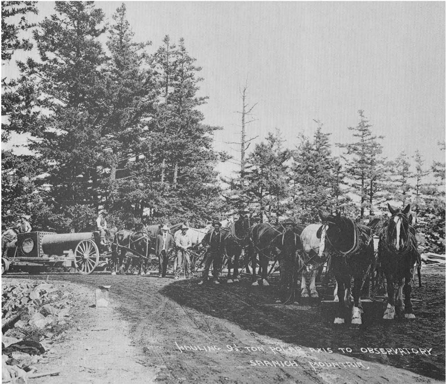
Hauling the nine and one-half ton polar axis up Saanich Mountain. National Archives of Canada. PA 149324.
