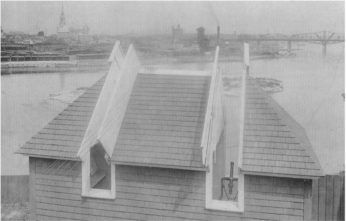
The transit house at the Cliff Street Observatory. National Archives of Canada, C 11614.
