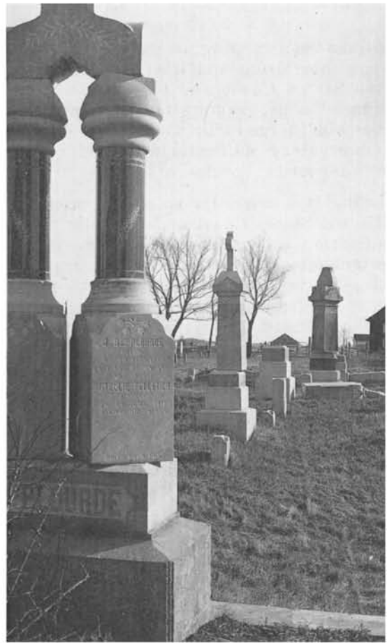
A row of tombstones; most of the distant ones have been tipped over, the one in the middle distance has shifted horizontally on its base, while the vertical pillars on the stone in the foreground have rotated.
