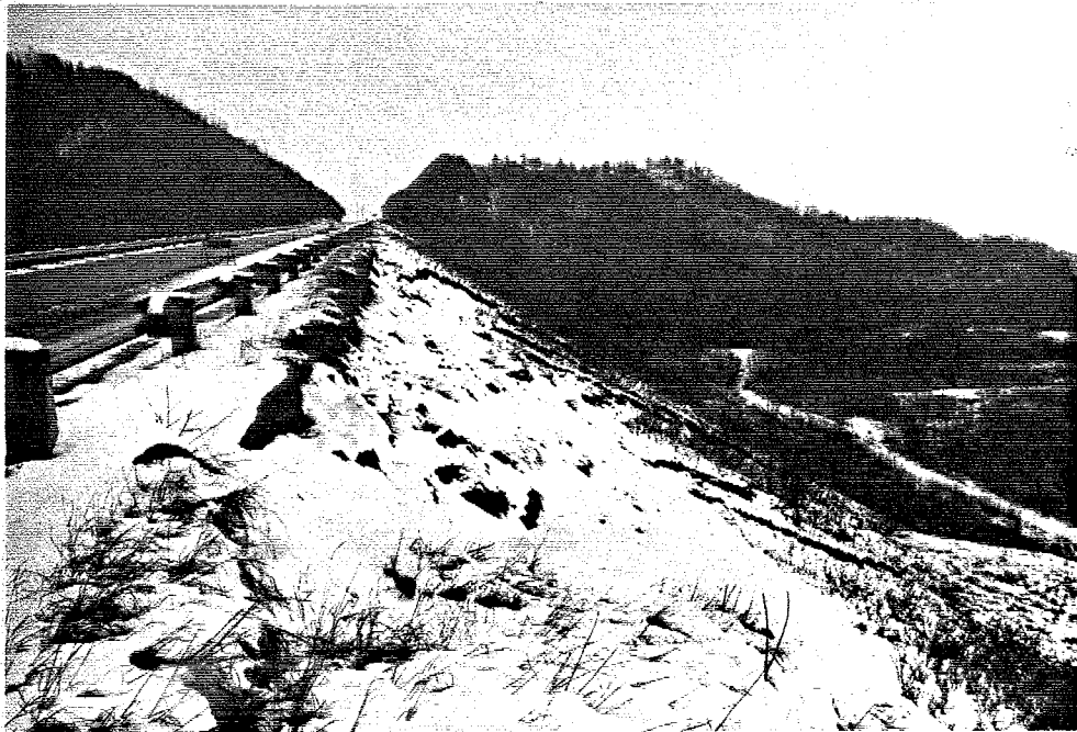
Figure 6.4 View of embankment failure from shoulder of highway.
