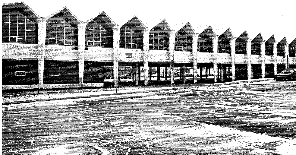
Figure 3.17 Overall view of Ecole Georges Vanier.
