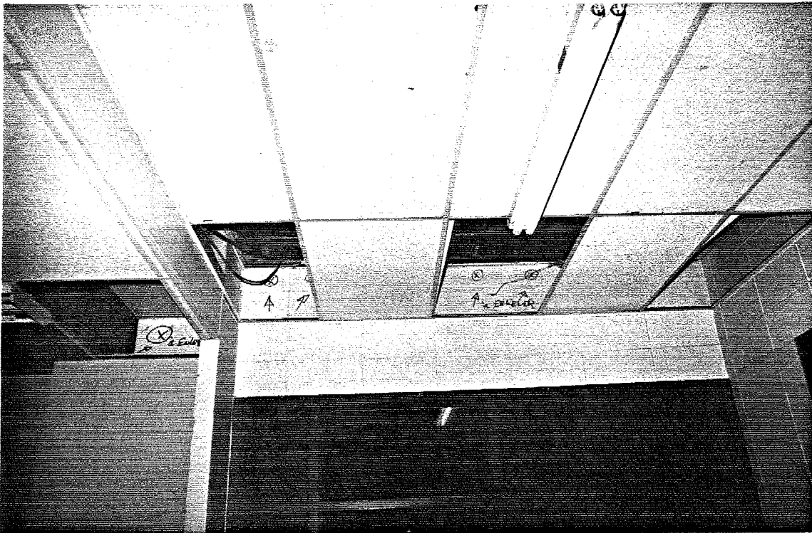
Figure 2.16 Identification of blocks to be removed for safety.
