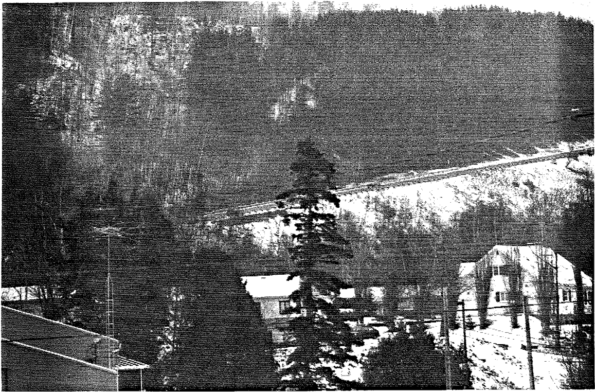
Figure 6.1 Location of embankment failure on Highway 138 near Ste. Anne de Beupré.
