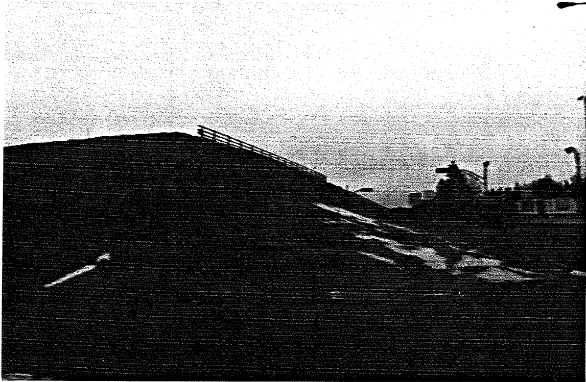
Figure 2.38 Well compacted sand fill embankment near Boulevard Talbot.
