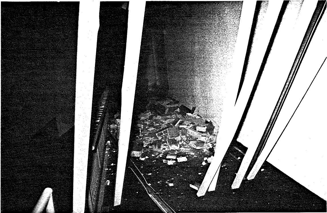
Figure 2.18 Debris from fallen masonry blocks in Dominique Racine school.
