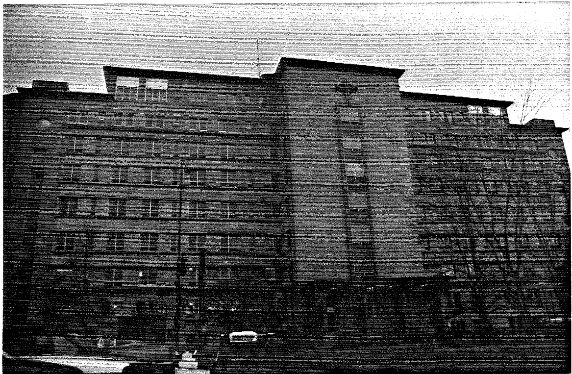
Figure 4.6 Wing B of Saint-François d'Assise Hospital.
