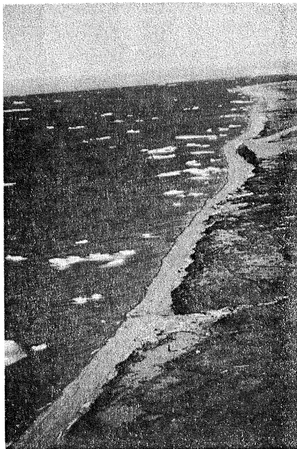
Figure 5.4 Photograph of low tundra cliffs at Komakuk Beach, Y.T. These cliffs are common in areas of the Tuktoyaktuk Peninsula in locally in other sections of the coast.
