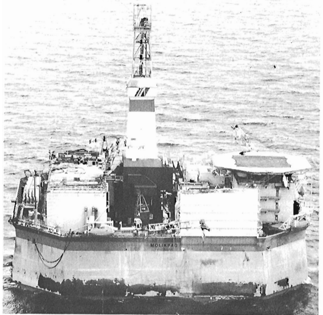
Figure 2. The Molikpaq, the mobile arctic caisson of Gulf Canada Resources from which the geotechnical corehole was drilled.
