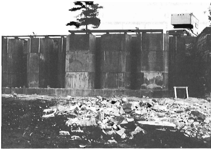
Figure 3.13. The nine concrete test columns at Bells Corners viewed from inside the quarry showing the "ore zones" and a logging truck parked above in the working area for calibrating logging systems. (GSC 203254-0).
