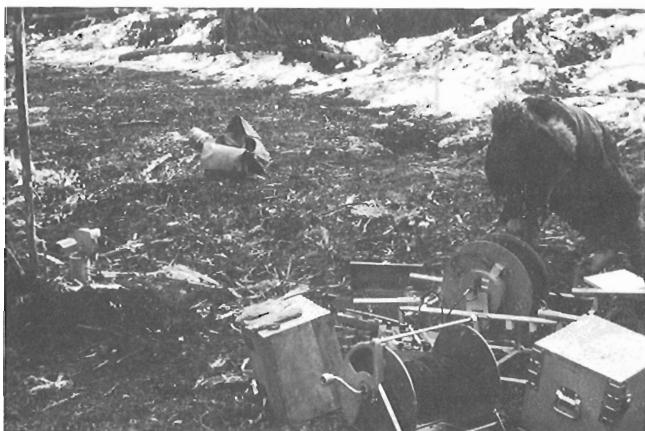
Figure 2. Crone DHPEM draw works (winch assembly).
