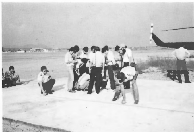
Figure 23. Painting a line on the pads to locate the helicopter skid.
