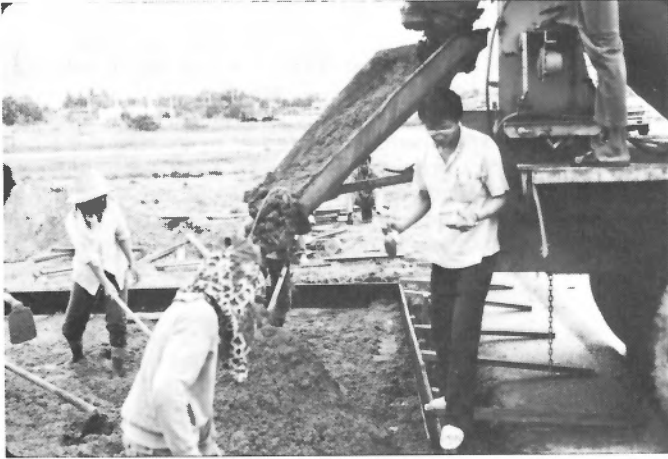
Figure 19. Sampling the sand-cement mix as it was being poured.
