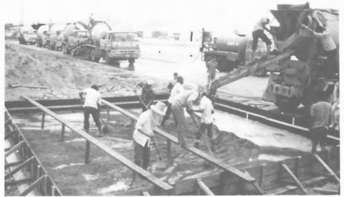
Figure 14. The pouring of the pads showing the wooden forms.
