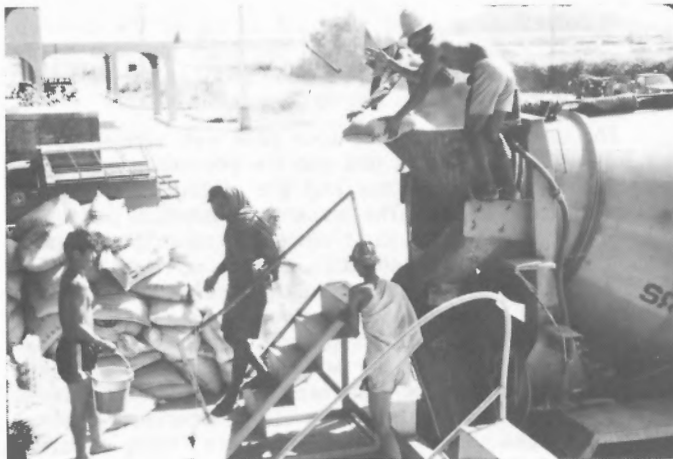
Figure 13. Loading a bag of sand into a cement truck.
