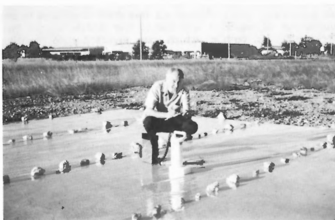
Figure 21. Sealing the uranium pad with a plastic sheet.
