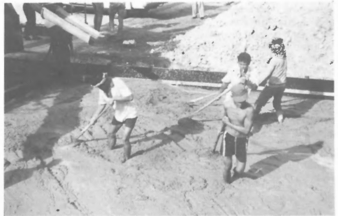
Figure 15. Spreading the sand-cement mix across the pad.
