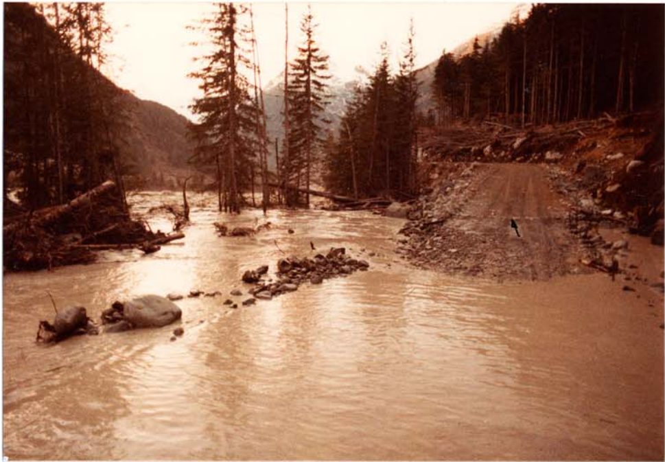
PL VIII A. Noeick River in flood at 1800 hrs. (Oct. 20, 1984) looking downstream from uppermost road washout. Note the turbulence of floodwaters in the middle channel (left centre) and stone line on the road (arrow) showing an earlier high water level. K.P. 34.6 Photo: K. Danielson
