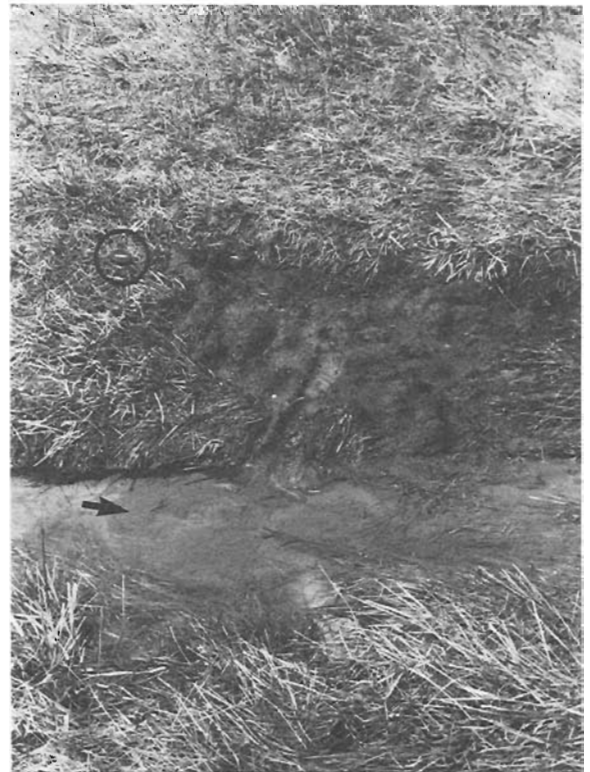
Figure 3. Molehill with a central tunnel that has become a seepage route. A small delta or fan (arrow) has formed downslope of the hill. The lens cap to the left of the molehill gives scale.
