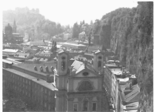
Figure 129: Southward view along the vertical Mönchsberg wall in the city centre of Salzburg. St. Marcus church in the foreground; festival theatre and castle in the background; note apartment buildings at the base of the cliff. (GSC 204167-C)
