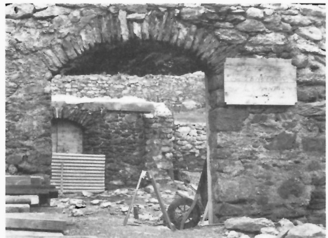
Figure 150: Recently excavated and renovated building foundations at the apex of the Nant Brun Torrent cone; note two generations of walls on the far side of the building. (GSC 204167-N)
