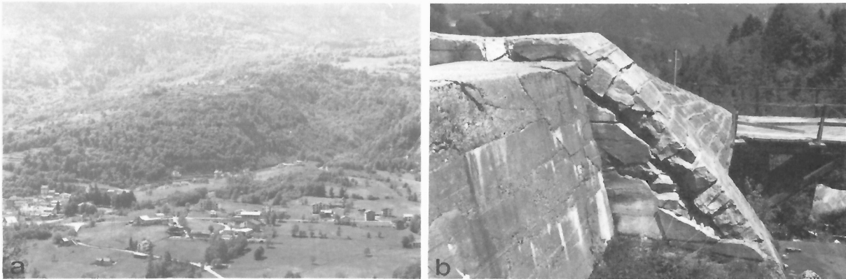
Figure 198: a) View of the Alfenza cone; village of Crodo on the left; note densely forested slopes bordering the Alfenza gorge and relatively new residential buildings along the formerly avoided central sector of the debris cone (GSC 204168-M). b) Damaged wing of a check dam in the upper Alfenza Torrent; the structure is being crushed by lateral stresses exerted by the sagging slope (GSC 204168-N).
