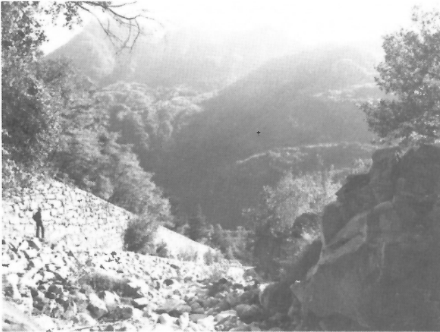
Figure 16: Debris deflection dam with strong stone-block armour (near Chiavenna, Italy). (GSC 204165-D)
