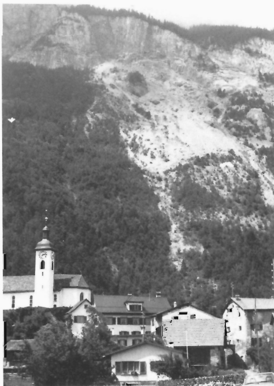
Figure 194: View of Felsberg-Altdorf and the carbonate dip slope behind the village; the church rests on a prehistorical slide block. (GSC 204168-K)
