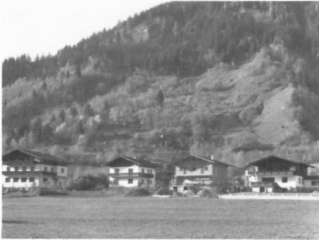
Figure 99: Typical slump in low grade metamorphic rocks of the Gastein region; note recently constructed tourist accommodations near the toe of the slide (GSC 204166-O).
