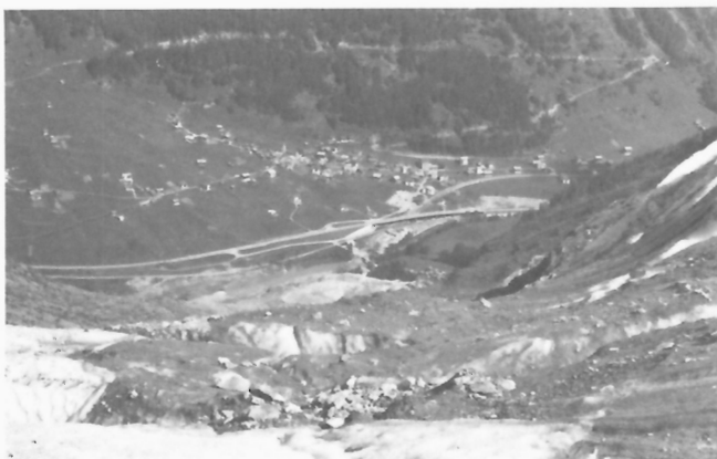
Figure 119: View of the Dorfbach cone and the community of Randa from the snout of the Bis Glacier; note several residential buildings near the axis of the cone in the runout zone of potential ice avalanches (GSC 204166-W).
