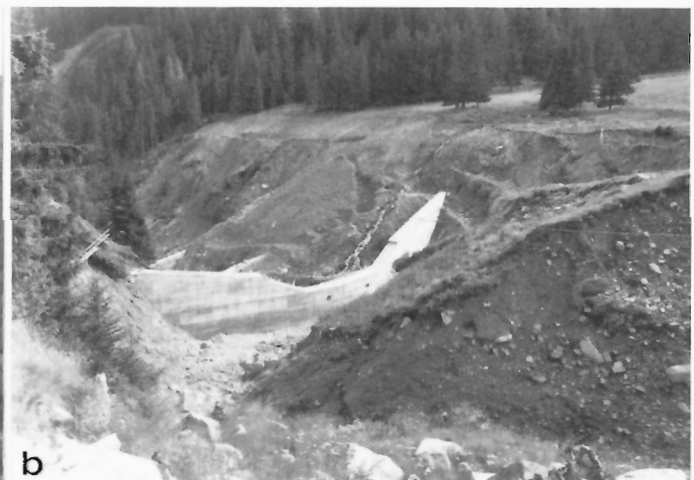
Figure 285: a) View of the crest of the Enterbach basin; note converging erosional ravines (GSC 204170-F). b) Steel-concrete check dam under construction on the Enterbach Torrent; note gently rising wings, deeply founded abutments, and drainage bores (GSC 204170-G).
