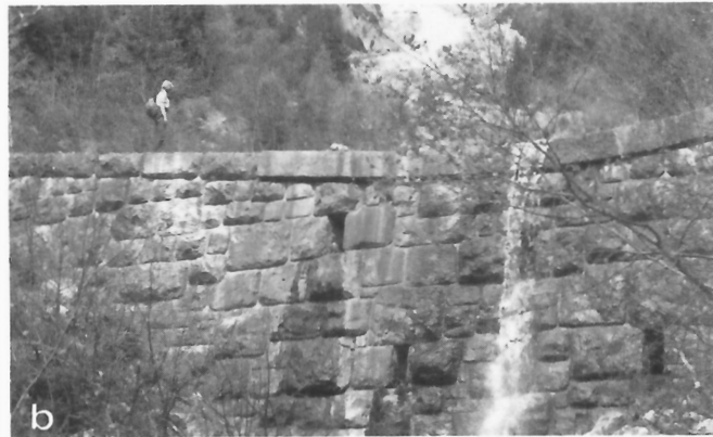
Figure 251: a) View of the intensely fractured carbonate cliffs near the summit of the Raucheck Massif; note the sparsely vegetated track of the 1947 debris flow in the ravine below the cliff (GSC 204169-L). b) Stone-masonry check dam across the upper Kammerloch Torrent built to prevent mobilization of carbonate rubble derived from the Raucheck Massif (GSC 204169-M).
