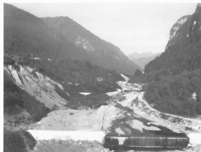
Figure 187: Northwestward view along the floodplain of the Vanoi Torrent at the toe of the Rebrutt cone (on the left); note wide-winged check dams designed to localize bedload transport and impede channel migration. (GSC 204168-F)
