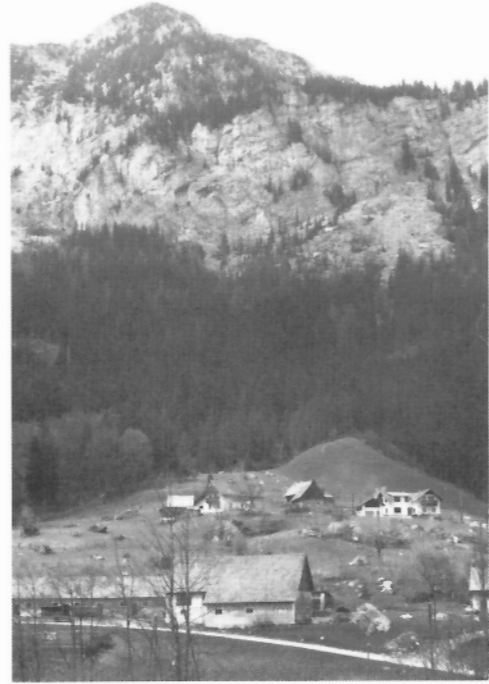
Figure 91: View of the western half of the built-over rock avalanche lobe at Radmer an der Hasel; note the thoroughly shattered bedrock spur overlapped by fresh rockfall debris and the flanks of the historical detachment zone on the west (left background) (GSC 204166-J).
