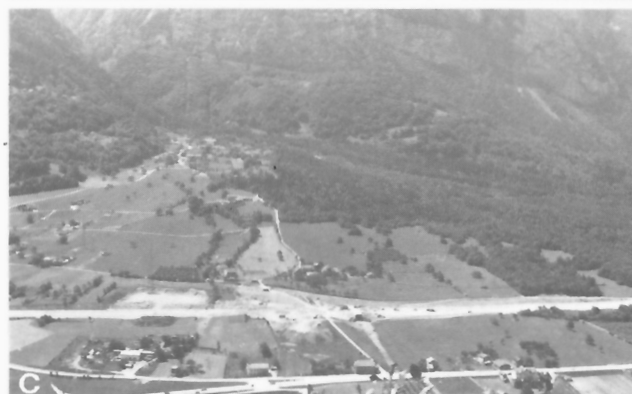
Figure 201: a) View towards the rugged summit ridge of the Dents du Midi from the top of the Gorge du Foillet; note large masonry check dam built in the 1930s (GSC 204168-O). b) Recently completed steel-concrete dam across the Gorge du Foillet; note temporarily impounded snowmelt runoff behind the structure (photograph taken in 1981) (GSC 204168-P). c) View across the Bois Noir cone; note protective pine forest on the northern sector of the cone (right); farms and residences dot the southern sector (GSC 204168-Q).
