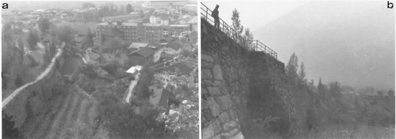
Figure 143: Two views of the protective debris deflection dam between the channel of the Schladraun Torrent and the modern buildings of Schlanders. (a. GSC 204167-K, b. GSC 204167-L)
