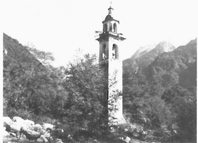
Figure 111: Church tower projecting from lobes of gneissic rubble on the cone of the Carmezzano Torrent. (GSC 204166-S)
