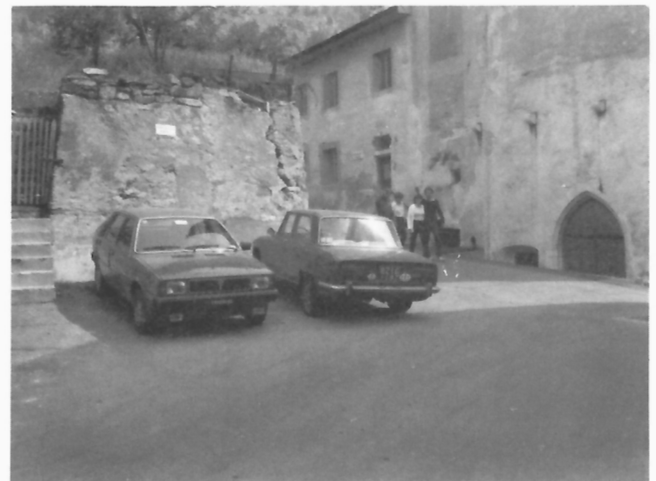
Figure 142: View of the church entrance below street level at Schlanders, indicating the incomplete excavation effort after the catastrophe of 1731. The height of the wall on the left indicates roughly the depth to which the town was buried in 1731. (GSC 204167-J)
