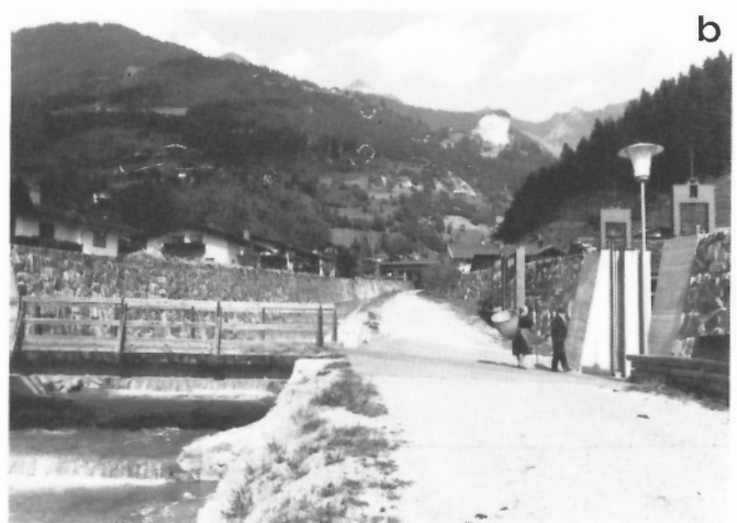
Figure 93: a) Concrete-masonry check dams spanning the lower part of the Bretterwandbach gorge above Matrei (person on the lower left for scale). Dense alder growth attests to present channel stability. In the background is a leaning limestone cliff forming part of the sagging Glunzerberg (GSC 204166-K). b) Protective masonry-concrete dykes flanking the Bretterwandbach channel in Matrei. The bridge can be raised mechanically during times of heavy runoff or threatening debris flows (GSC 204166-L).
