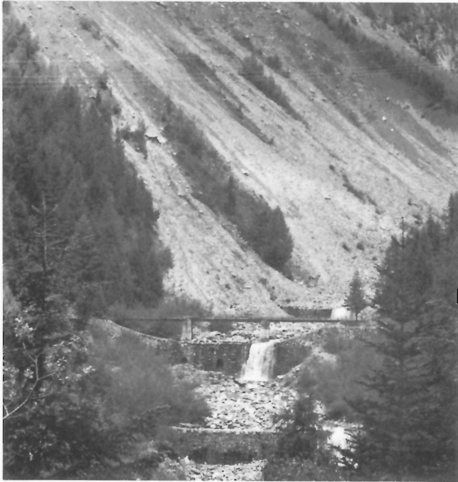
Figure 215: Masonry check dams along the rubbly toe of the Bec Rouge slide; check dams have prevented the torrent from eroding the loose landslide deposits. (GSC 204168-X)
