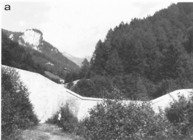
Figure 93: a) Concrete-masonry check dams spanning the lower part of the Bretterwandbach gorge above Matrei (person on the lower left for scale). Dense alder growth attests to present channel stability. In the background is a leaning limestone cliff forming part of the sagging Glunzerberg (GSC 204166-K). b) Protective masonry-concrete dykes flanking the Bretterwandbach channel in Matrei. The bridge can be raised mechanically during times of heavy runoff or threatening debris flows (GSC 204166-L).
