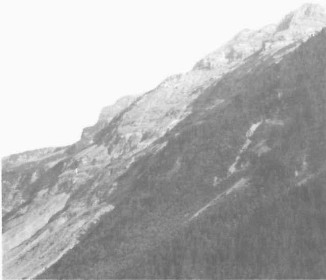
Figure 223: Detachment zone of the Spitzen rockslide; failure occurred along a stepped composite fracture surface cutting across the bedding. (GSC 204169-C)
