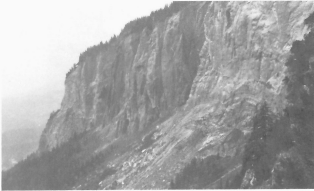
Figure 249: View westward along the steep carbonate cliff of the Flimserstein above Fidaz. (GSC 204169-K)
