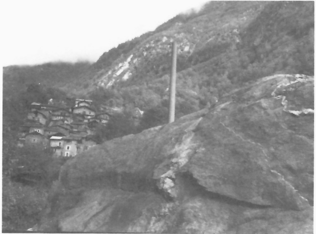
Figure 192: Steep rockfall cone and part of Spriana. (GSC 204168-J)
