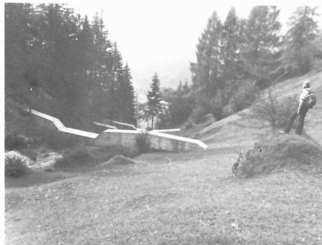
Figure 274: Recently completed array of check dams across a ravine above Siror which is carved into slump-prone relict colluvium and phyllitic bedrock. (GSC 204170-A)
