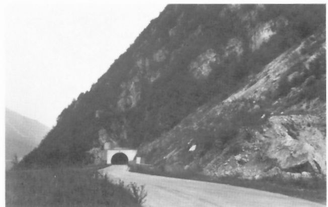
Figure 57: View to the north along the shore of Lago di Santa Croce. A recent highway tunnel pierces the northern flank of the Fadalto slide scar following the strike of the dip slope in massive carbonate rock. (GSC 204165-P)
