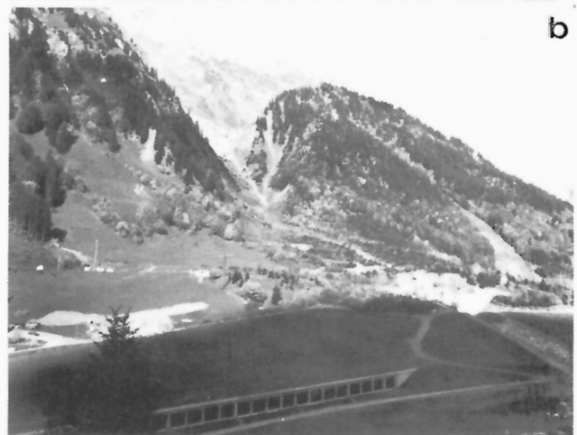
Figure 228: a) Photograph of the Blisadona rock avalanche shortly after the event (from Toula, 1893). b) The Blisadona cone today: a modern highway gallery pierces the debris cone and an armoured channel facilitates the passage of runoff, snow avalanches, and rare debris flows (GSC 204169-E).
