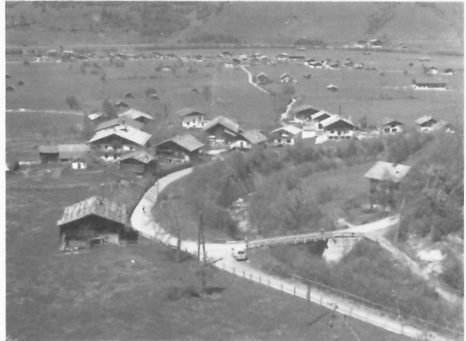
Figure 171: View of Mühlbach (foreground) and Niedernsill (background); note the sharply curved protective debris diversion dam and continuing construction activity on the upper fan. (GSC 204167-X)
