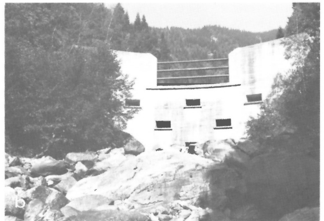
Figure 16: Debris deflection dam with strong stone-block armour (near Chiavenna, Italy). (GSC 204165-D)
