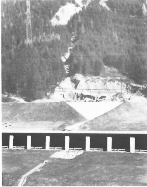
Figure 18: Combination of debris retention basin and gallery designed to protect major mountain highway from recurrent debris flows (Arlberg Highway, Austria). (GSC 204165-H)
