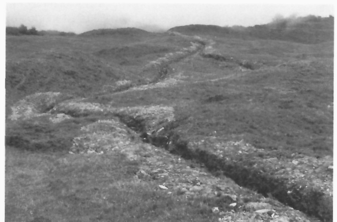
Figure 210: View of surface drainage ditches on the undulating upper part of the Heinzenberg slope; snowmelt runoff is thus prevented from accumulating in and infiltrating along sag ponds on the slope. (GSC 204168-U)
