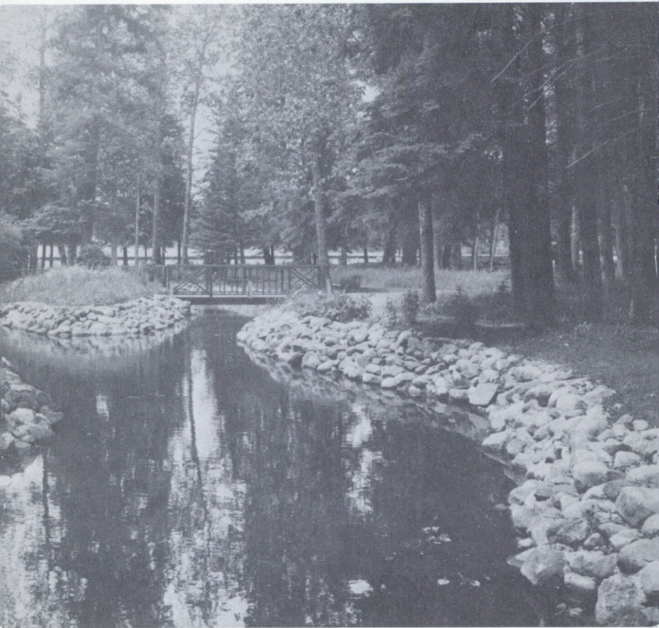
Retaining walls constructed of boulders.
