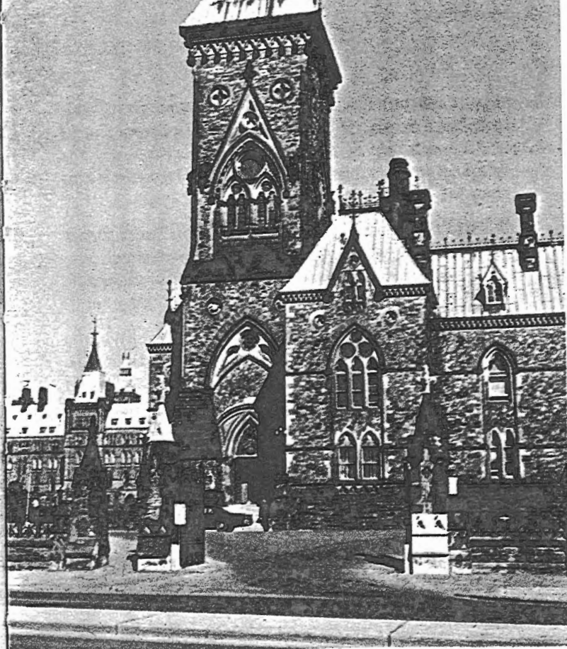
The East Block, part of the original Parliament Buildings built in the 1860's, shows a great variety of different stones on its south face. Nepean sandstone forms most of the walls, with trim in plain and carved blocks of Wallace sandstone (khaki). Red sandstone trim forms the arches and inset rosette with a variety of field stones used in potpourri above the door. The grey steps are limestone.
