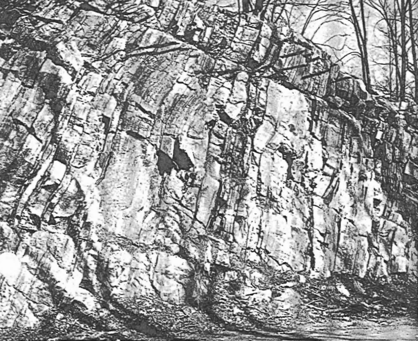
Ottawa Limestone tilted up on edge marks the trace of the fault system across McCarthy Road. Note the gently dipping or sloping surface of breakage near the top of the outcrop and the minor bending about half way up the cliff.
