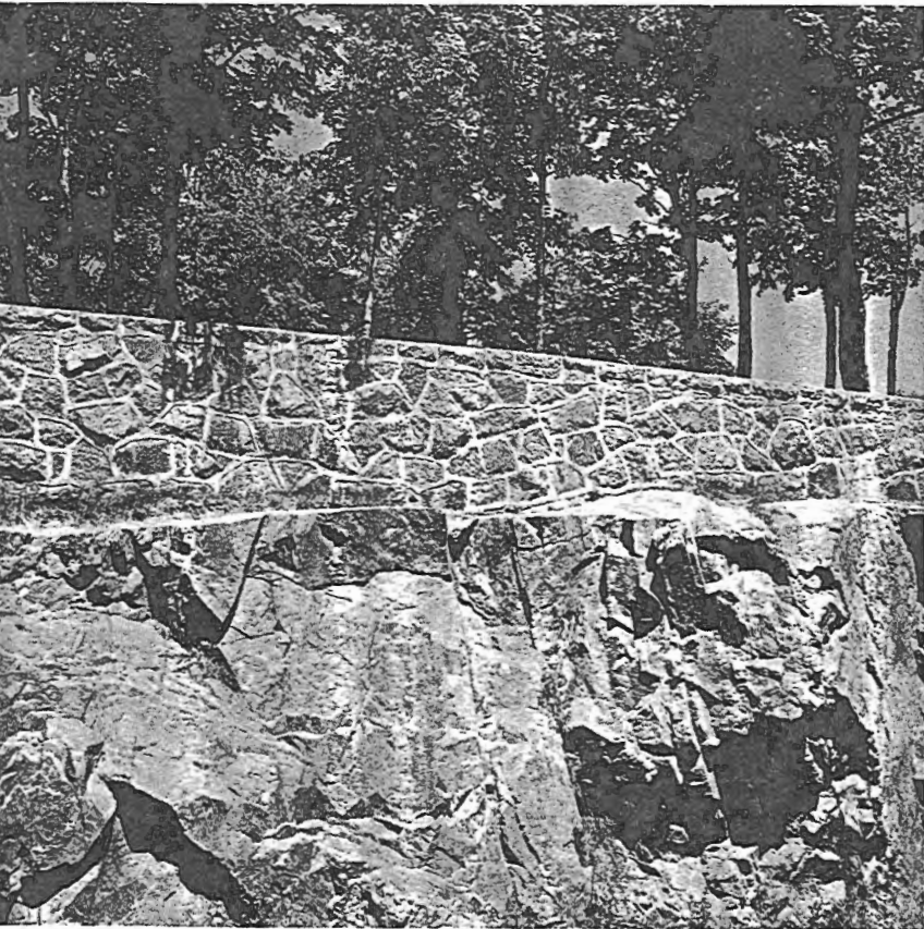
Retaining and decorative walls along the Gatineau Parkway, especially near the Champlain Lookout end, are built of stone imported from the Montreal area.
