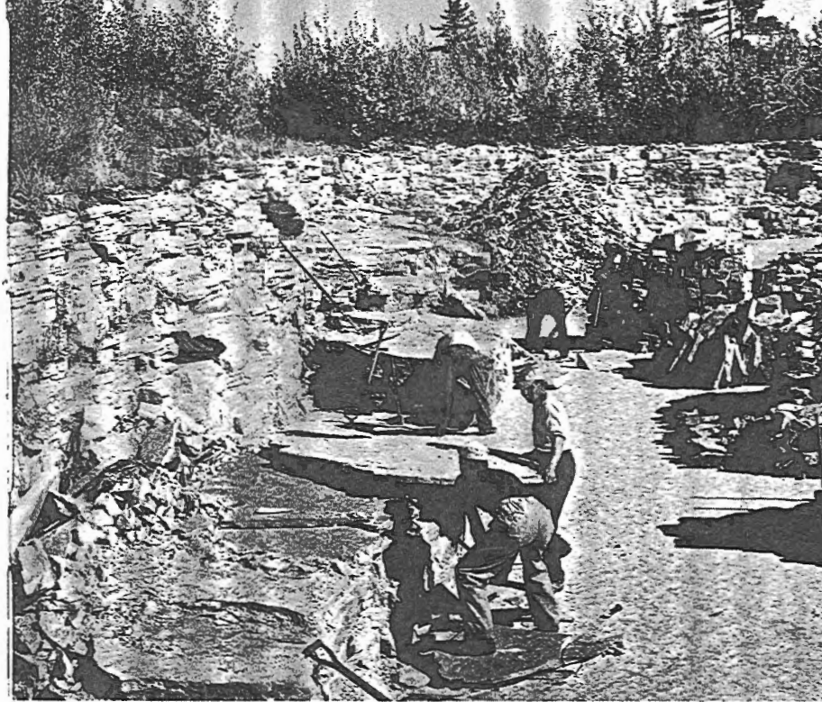
Removing flagstone and building stone from the Nepean sandstone outcrops at the old Campbell's quarry, west of Bells Corners.
