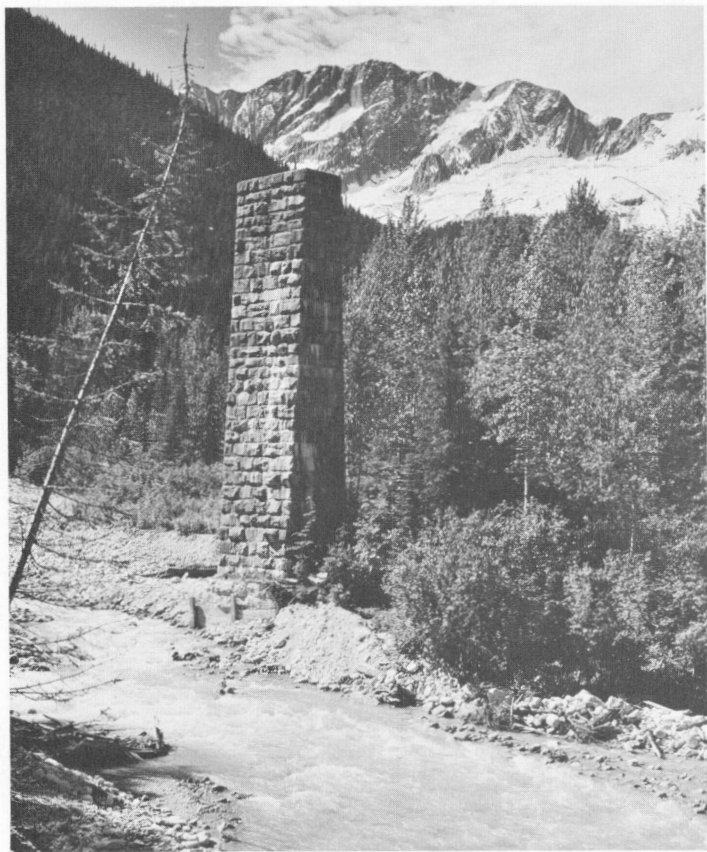
Bonney Névé (snowfield) lies high in the mountains beyond the foreground woods and the waters of Loop Brook. The tall masonry pylon used to carry the railway when it made a loop in this area to gain height in its former route through Rogers Pass.
