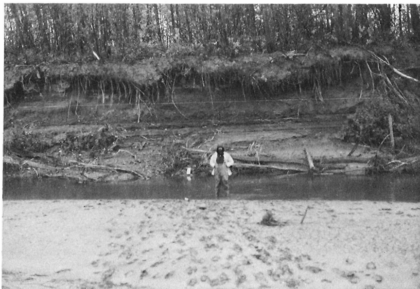
Figure 40.7. Photograph of eroding north bank of Steep Creek near the highway crossing. (GSC-203091)
