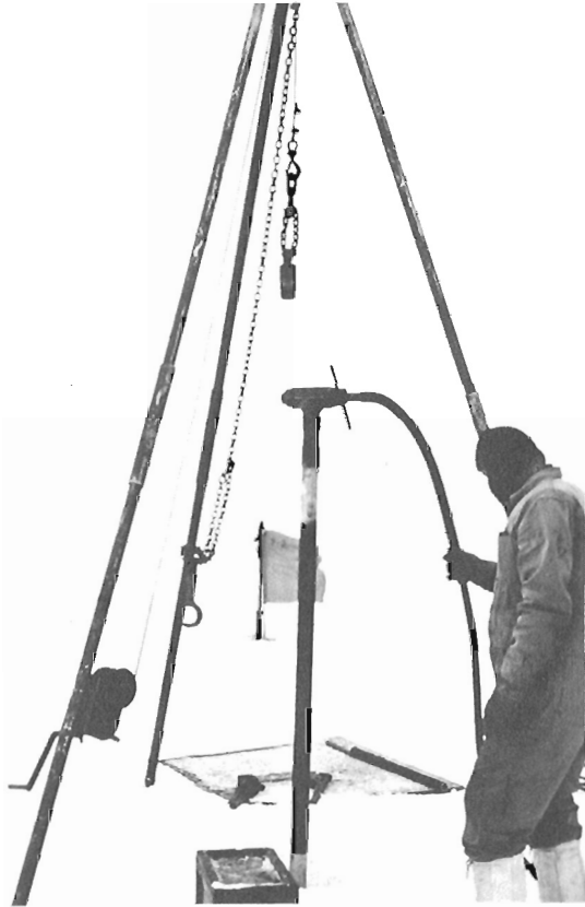
Figure 21.3. Tripod with winch assembly.
