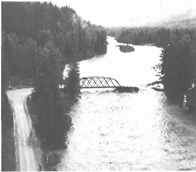
Figure 25.11. View up the Illecillewaet at Greeley, July 12, 1983 at approximate time of maximum discharge; note the partially destroyed bridge. (Photo courtesy of C. Macdonald, Water Survey of Canada)
