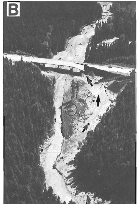
Figure 25.15. The partially destroyed Woolsey Creek bridge, Trans-Canada Highway, July 18, 1983. A – View to the west (GSC 204045-B). B – View down Woolsey Creek showing path of river flow (arrow) that undermined the west abutment. Note attempts to control Woolsey Creek (bulldozer circled) before construction of temporary crossing. (GSC 203993-X)
