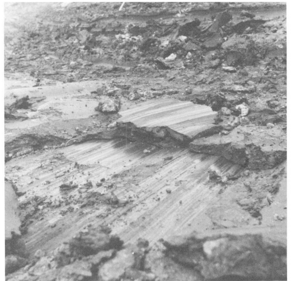
Figure 9. Large slickensides and fluting found on failure plane of Drynoch landslide. Failure plane was exposed in 1961 during construction activity. Photo by British Columbia Department of Highways.
