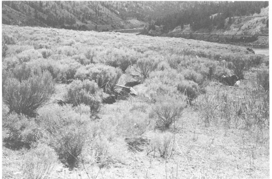
Figure 8. View looking south across the toe of Drynoch landslide showing tension crack of incipient toe failure. Shovel is 1.3 m long. Sage is typical of vegetation on lower portion of landslide. (GSC 175625)
