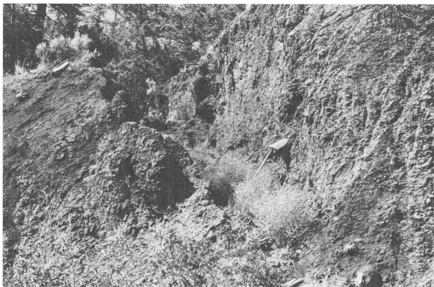
Figure 6. Large tension crack at break in slope of Drynoch landslide; the crack is 1.8 m wide and more than 3 m deep. (GSC 175637)
