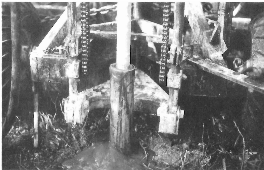
Figure 9.5. Gel used to seal cavities in bedrock. The semi-solid, stringy mass pouring out of the casing results from adding Borax solution to high viscosity Revert drilling fluid. 203506-G.
