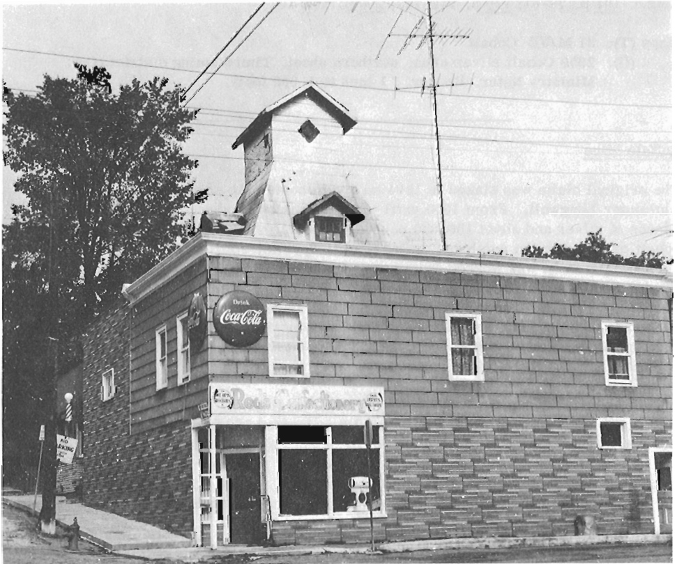
Plate V. Coniagas Mine, Shaft No. 4; the headframe has been enclosed within a local grocery store in Cobalt. (G. S. C. photo 161463)
