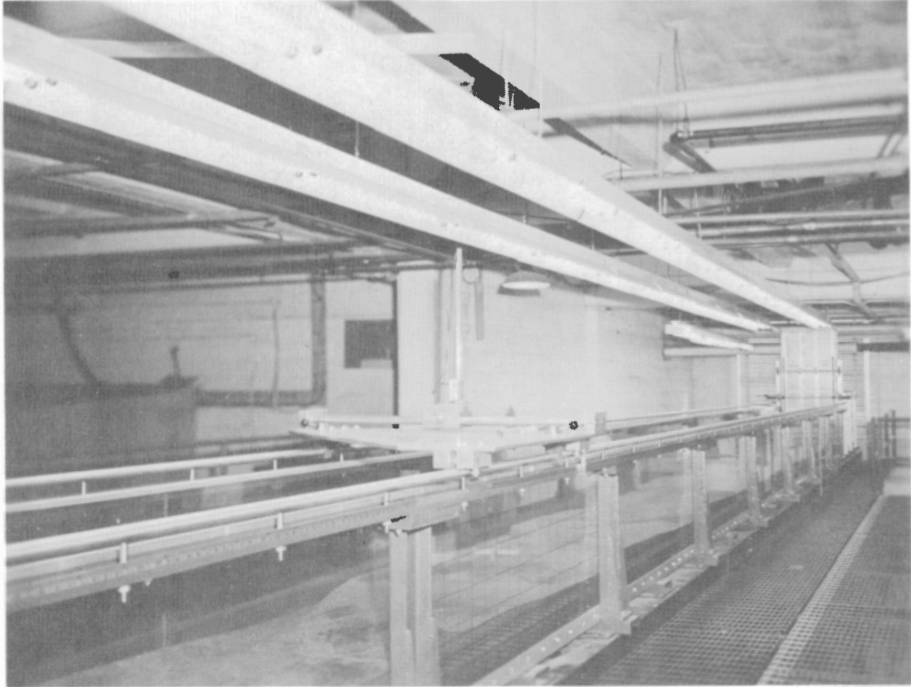
Figure 3. Main channel, looking upstream. GSC photo 201625-B
