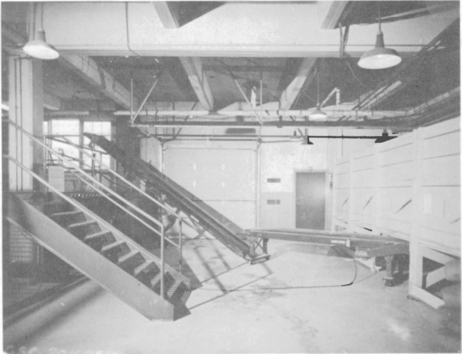
Figure 9. Sediment-storage bins with conveyor belts leading to tail tank. GSC 201625-C
